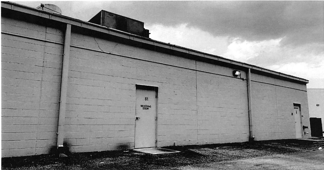
Source: Planning & Development Department, 08/11/2020
