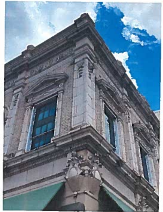
Photo 18-Exterior Facing South Along N. Laura Street
