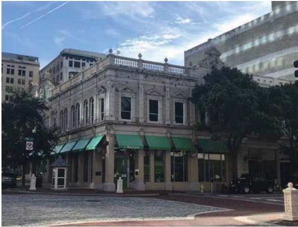
Figure 4-Current View of the Old Bisbee Building
