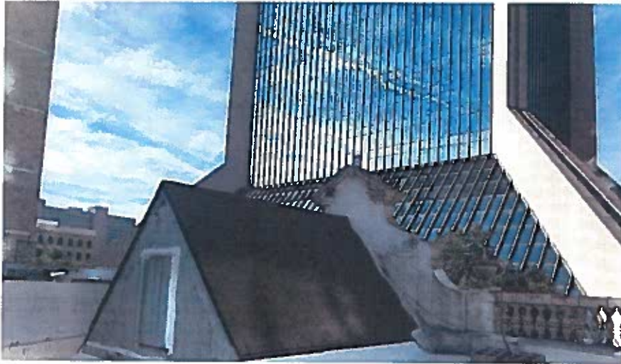
Photo 17-Rooftop View Facing W. Bay Street
