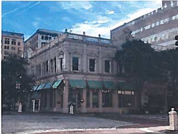
Figure 6-Current View of the Old Bisbee Building
