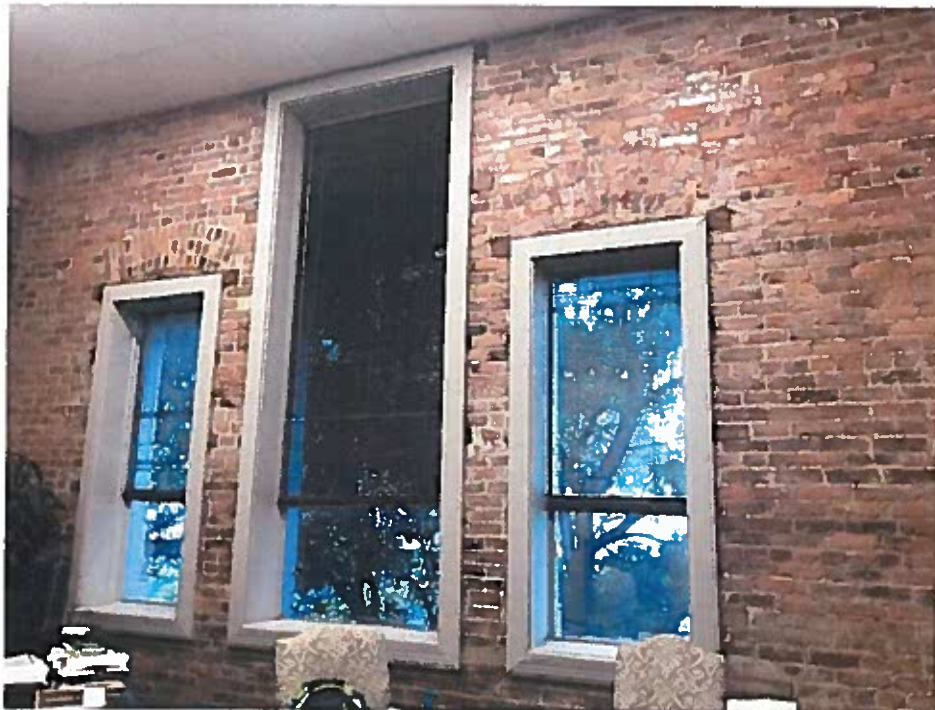
Photo 21-Interior of the Old Bisbee Building
