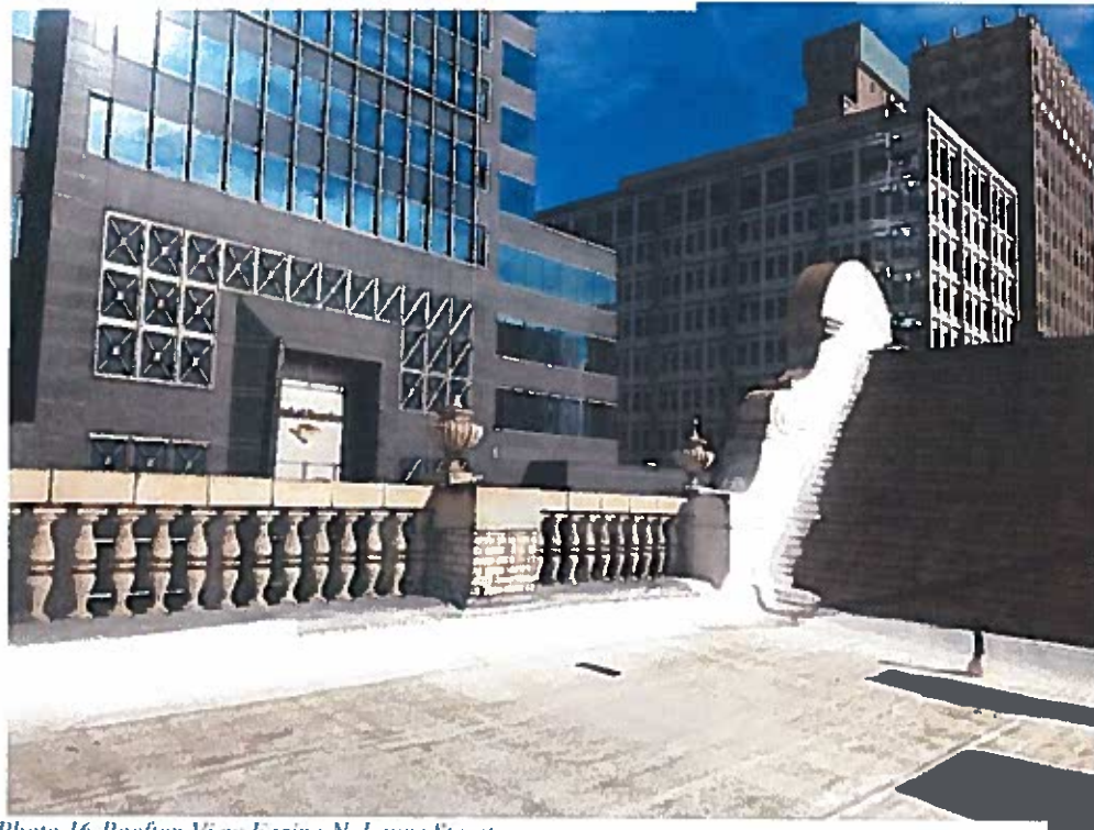
Photo 16-Rooftop View Facing N. Laura Street
