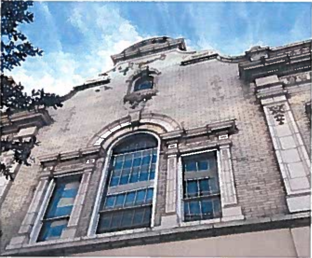
Photo 8-Most Northern Parapet Along N. Laura Street
