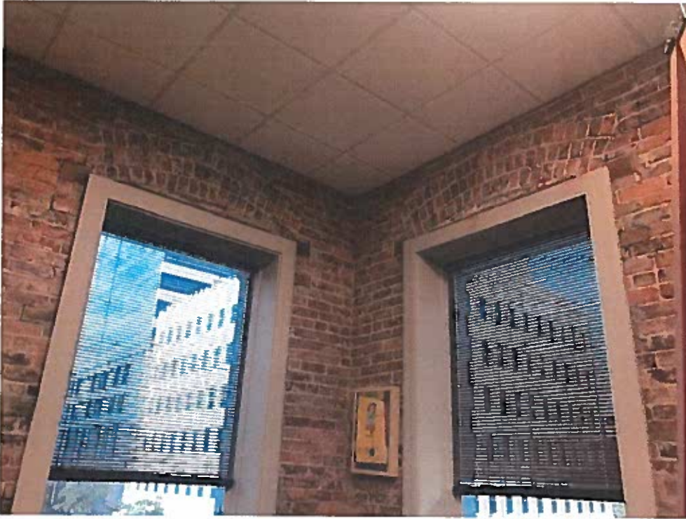
Photo 22-Interior of the Old Bisbee Building
