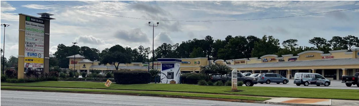
View of Shopping Center from San Jose Boulevard
