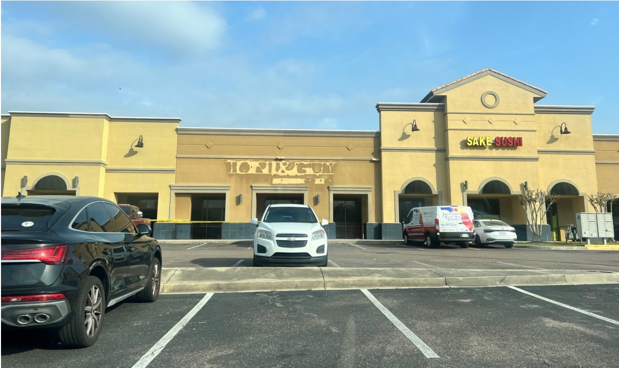
Source: Planning & Development Department, 3/24/25
