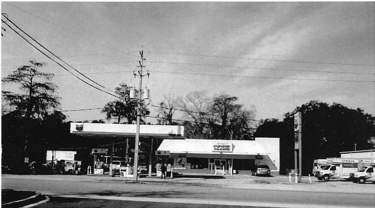
Property to the west: Gas Station
