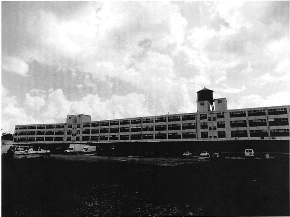
Photo 4 - Exterior, west façade (front), north end, looking east.
