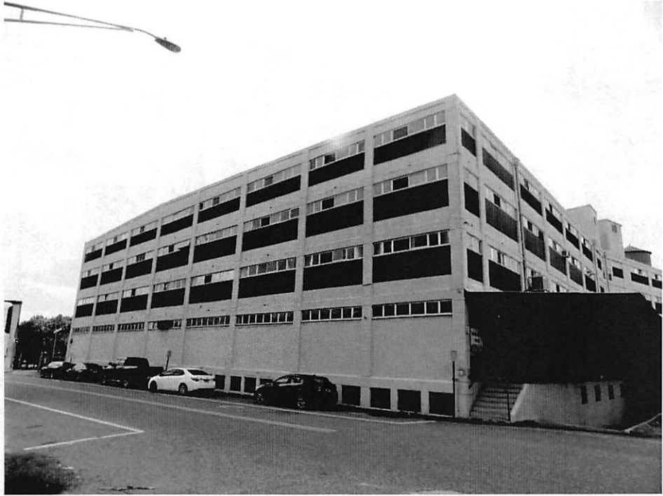
Photo 3 - Exterior, north façade along Union Street, looking southeast.
