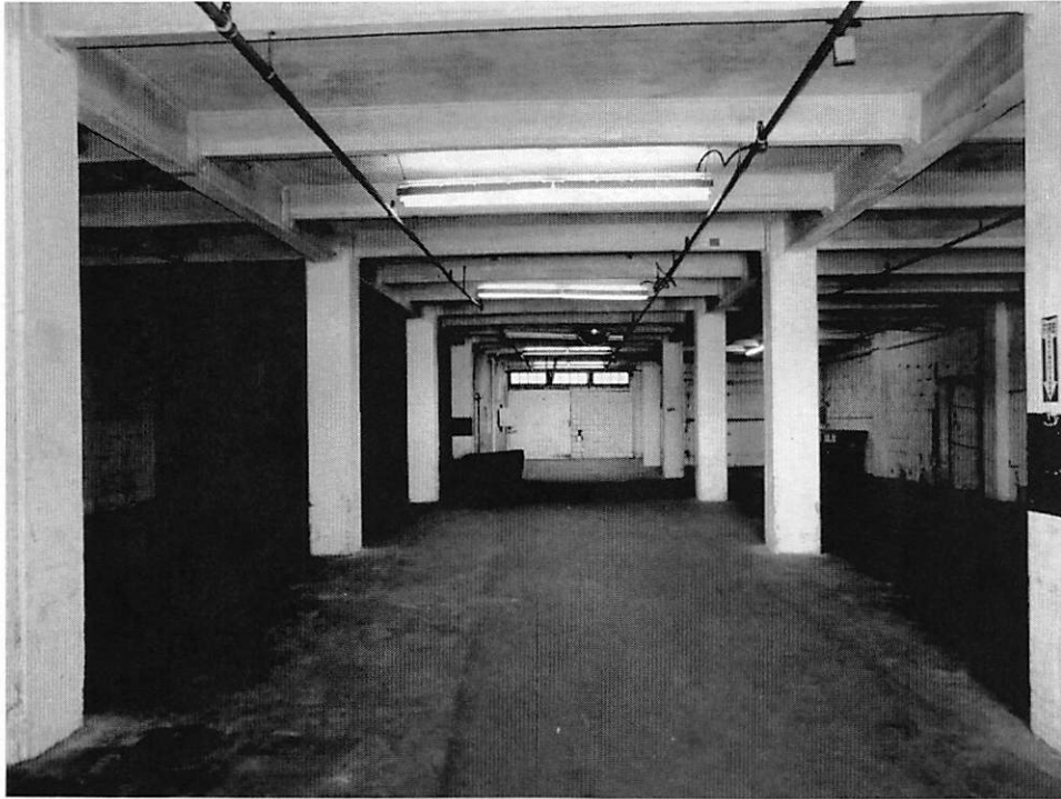
Photo 21 - Interior, first floor Unit D, looking east.
