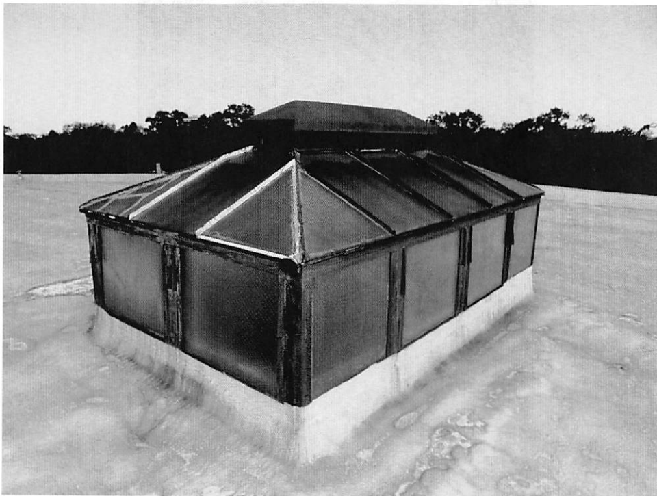
Photo 18 - Exterior, roof skylight, looking northwest.
