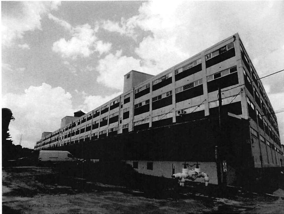
Photo 9 - Exterior, east façade, looking southeast.
