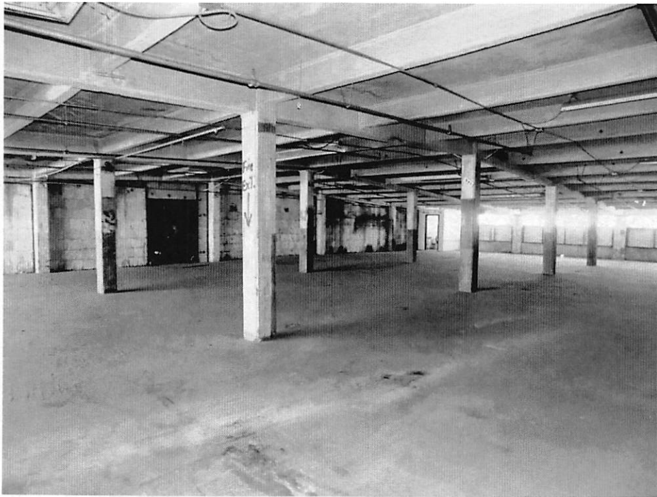
Photo 22 - Interior, fourth floor Unit E, looking southwest.
