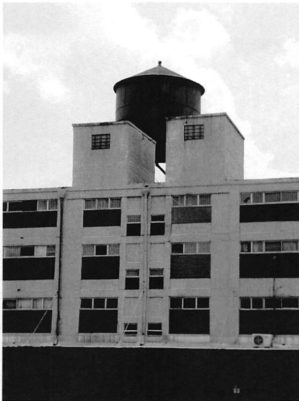
Photo 6 - Exterior, west façade (front), water tower and stair tower detail, looking east.
