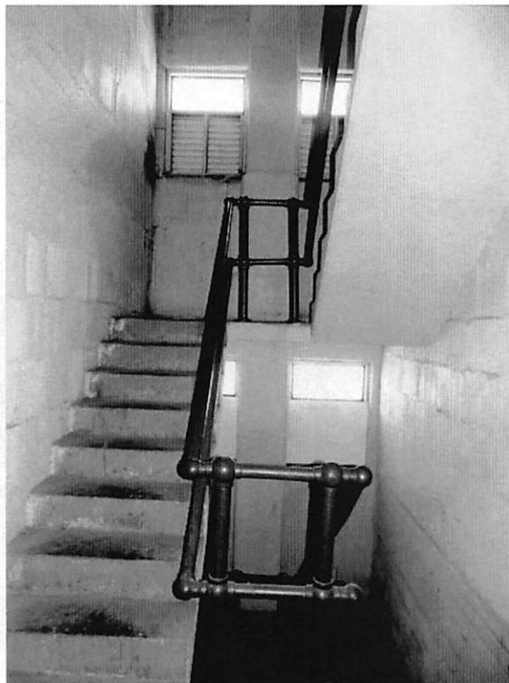
Photo 35 - Interior, third floor Units F and G, stairwell, looking west.
