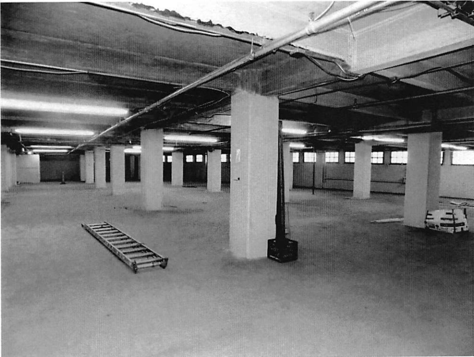
Photo 20 - Interior, basement Unit A, looking northwest.
