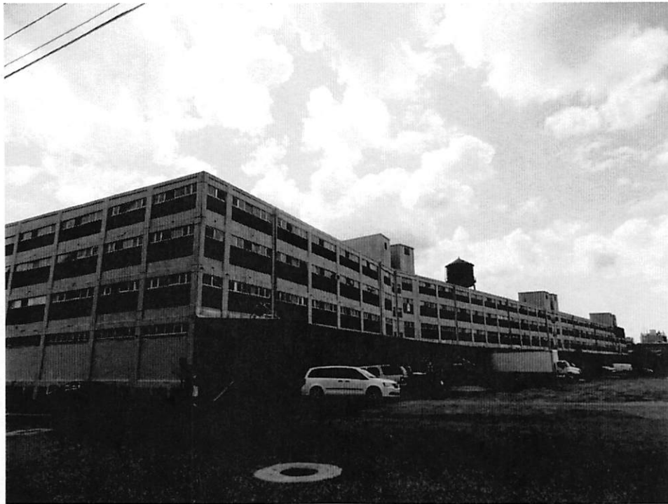
Photo 1 - Exterior, north and west (front) facades, looking southeast.
