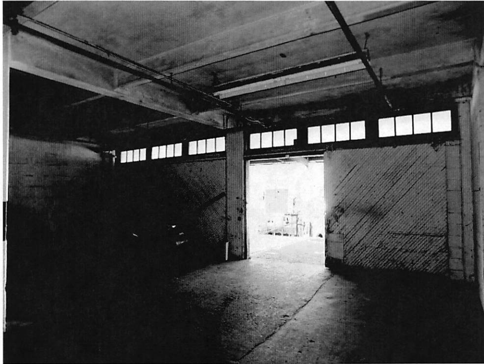
Photo 15 - Interior, first floor unit D, loading doors, looking southwest.
