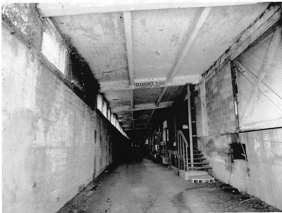
Photo 12 - Lower driveway on west façade (front), looking north.
