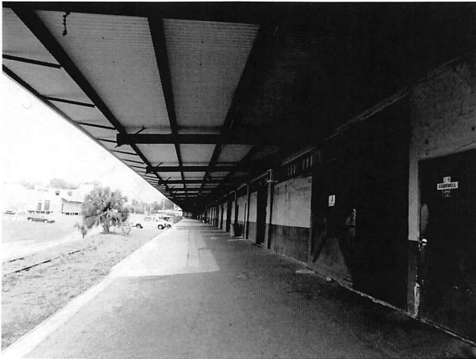
Photo 10 - Exterior, west façade (front), loading dock, looking north.
