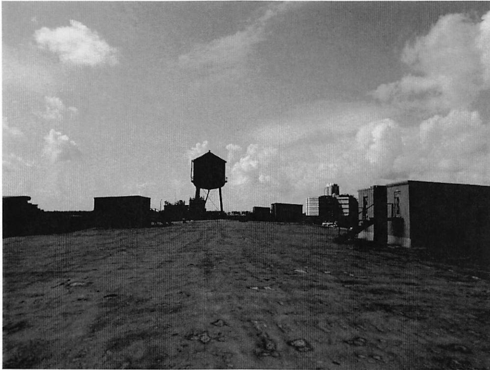
Photo 17 - Exterior, roof, looking south.
