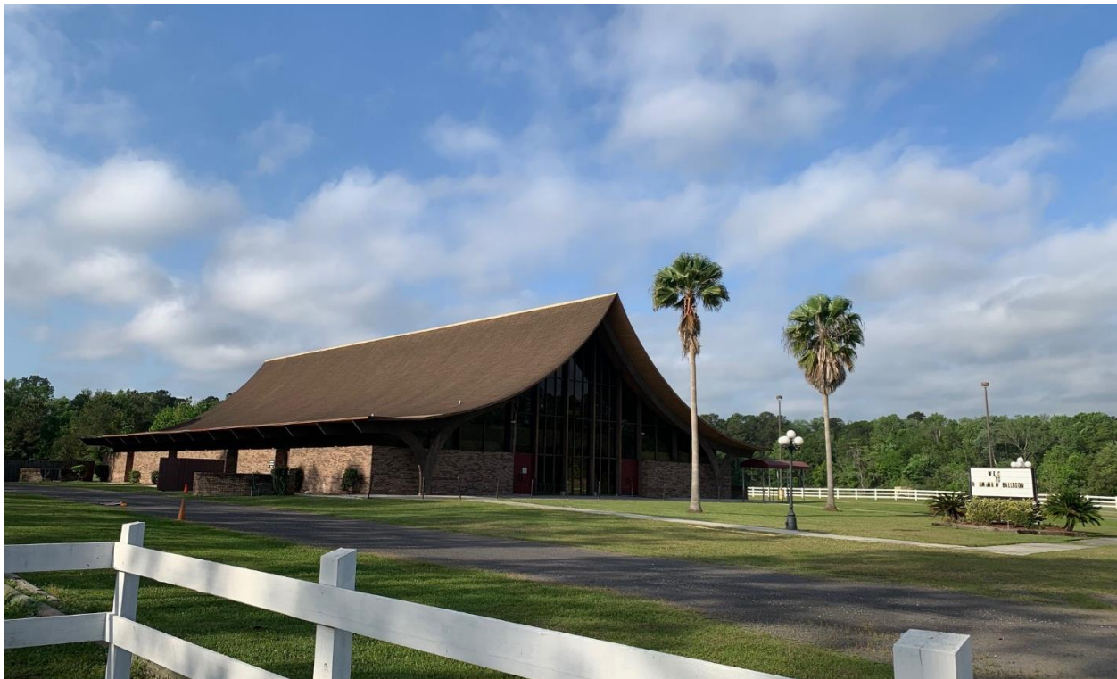
Source: Planning & Development Department, 3/26/2020
