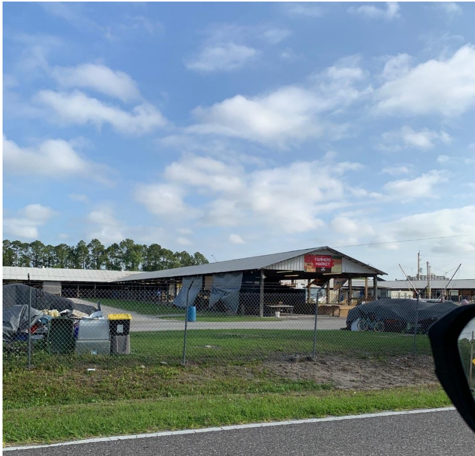
Source: Planning & Development Department, 3/26/2020
