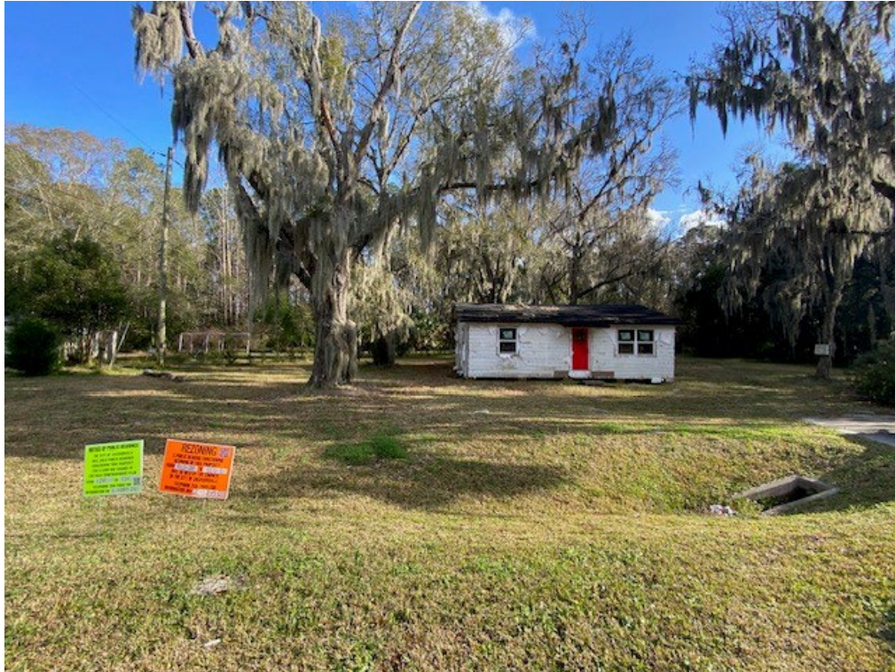
View of dwelling on subject property.
