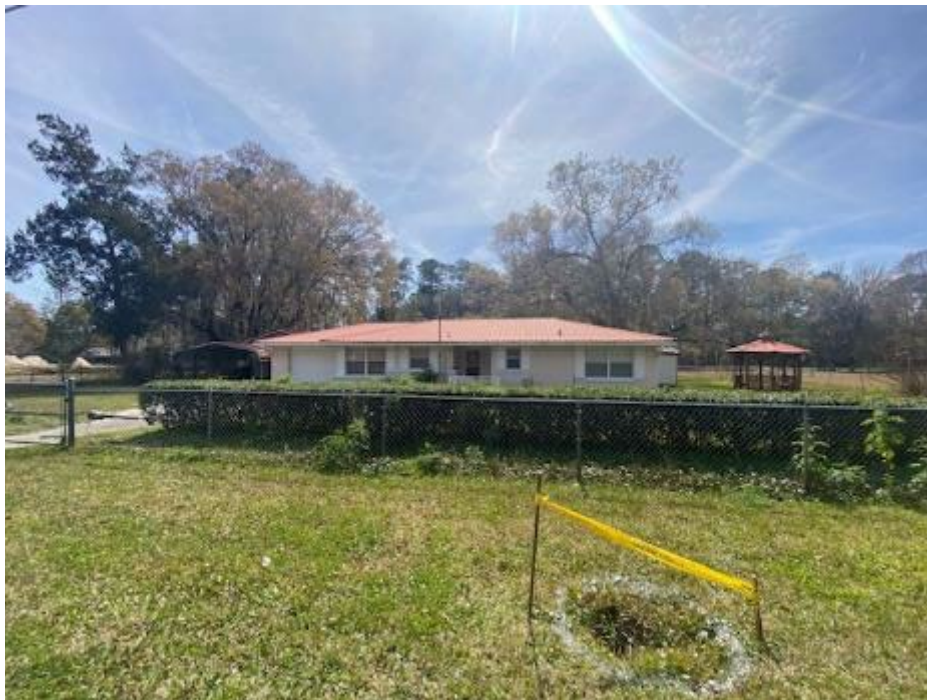
View of single family dwelling on the northern portion of the subject property.
