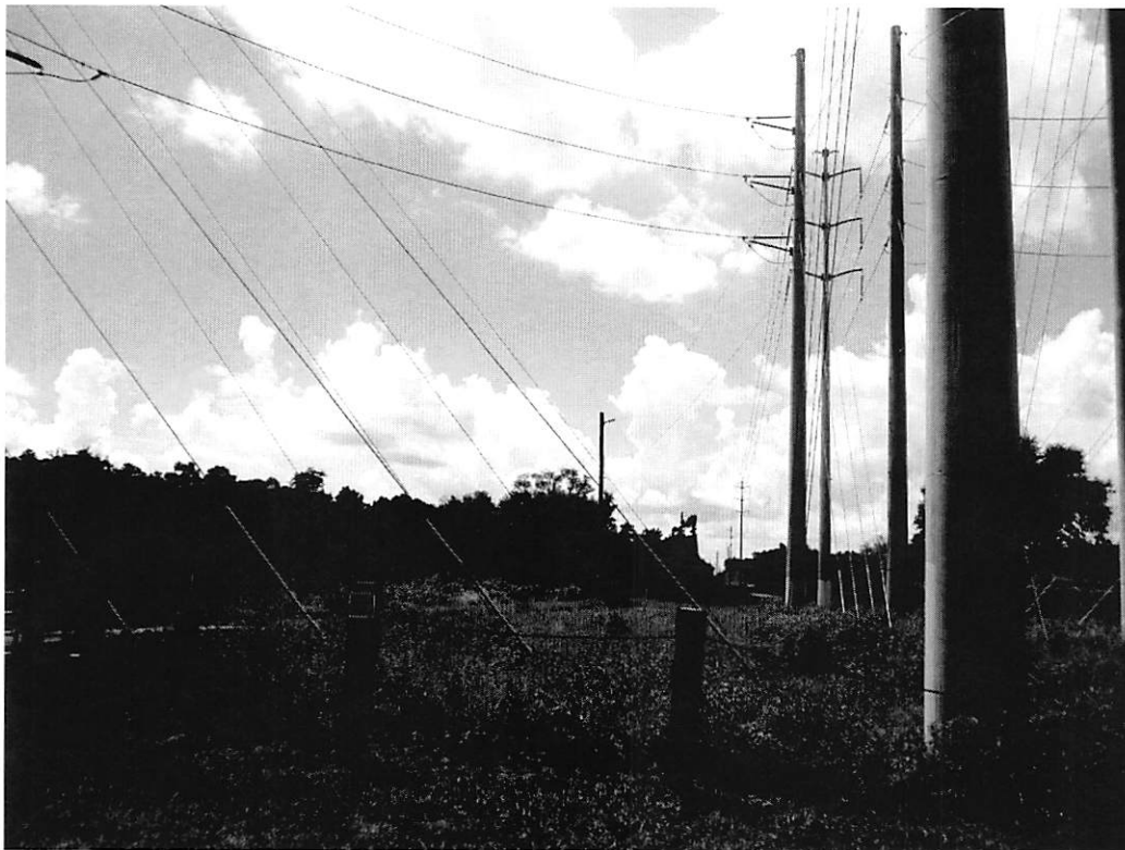
View of the Subject Site from the proposed entrance
