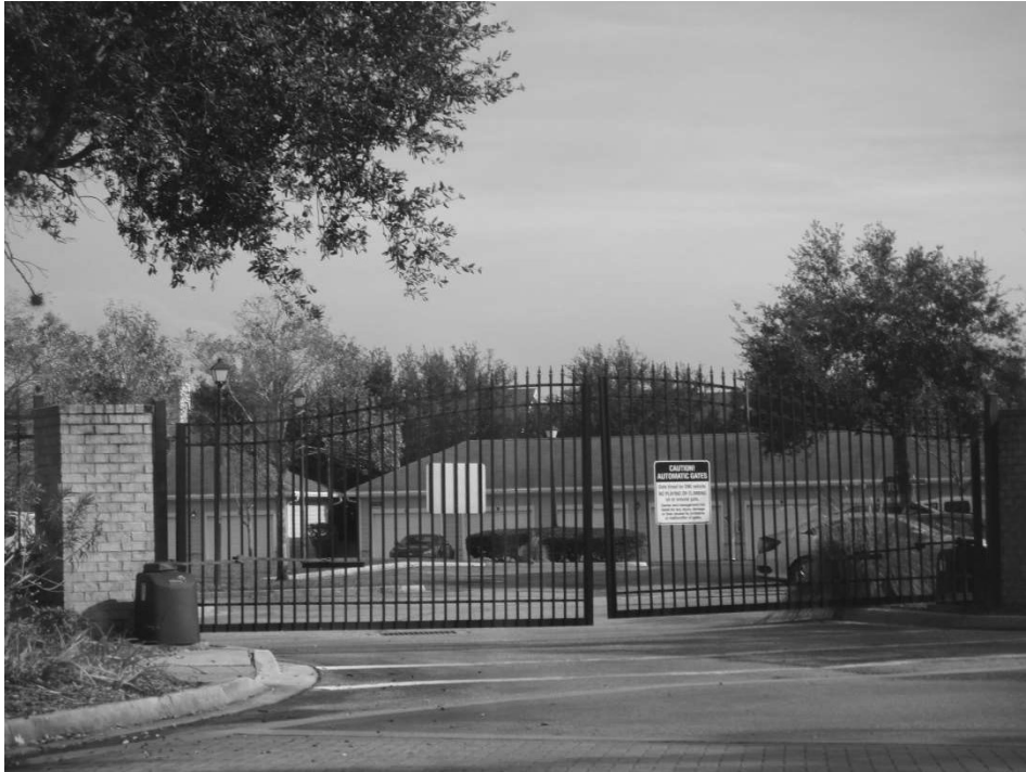
View of the existing Garage Structures on the Subject Site
