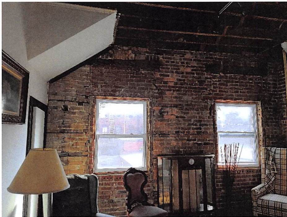
Photo 10, original brick exposed on interior
