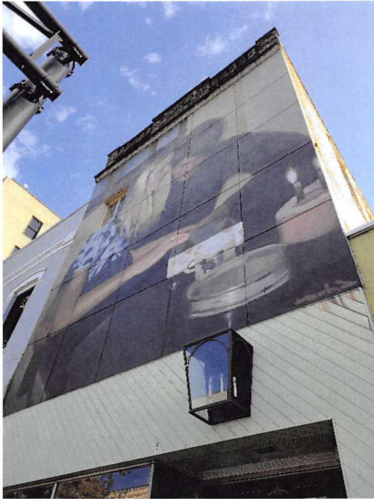
Photo 6, stucco panels with mural
