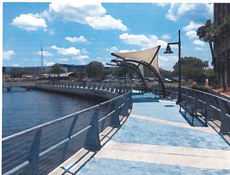
Existing Southbank Riverwalk railing and materials.
