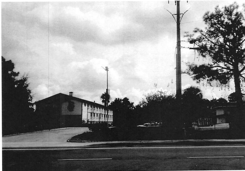
Property to the south of eastern subject property: Motel
