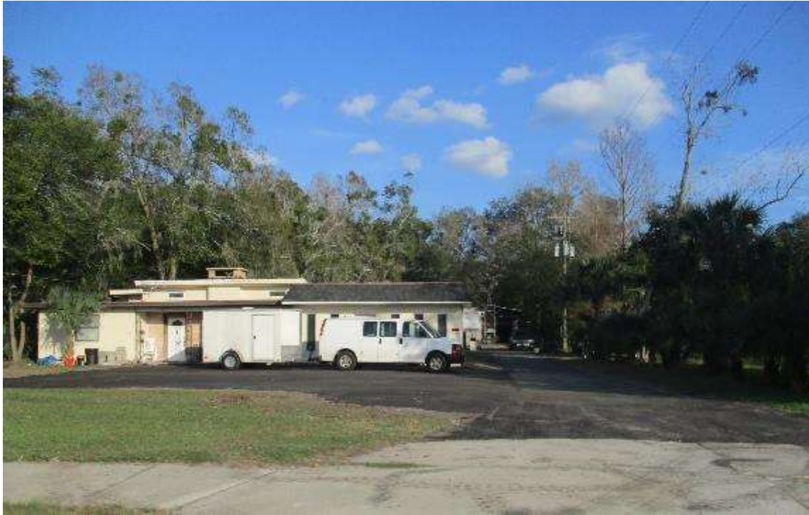
Office building across Wesconnett Blvd from subject property
