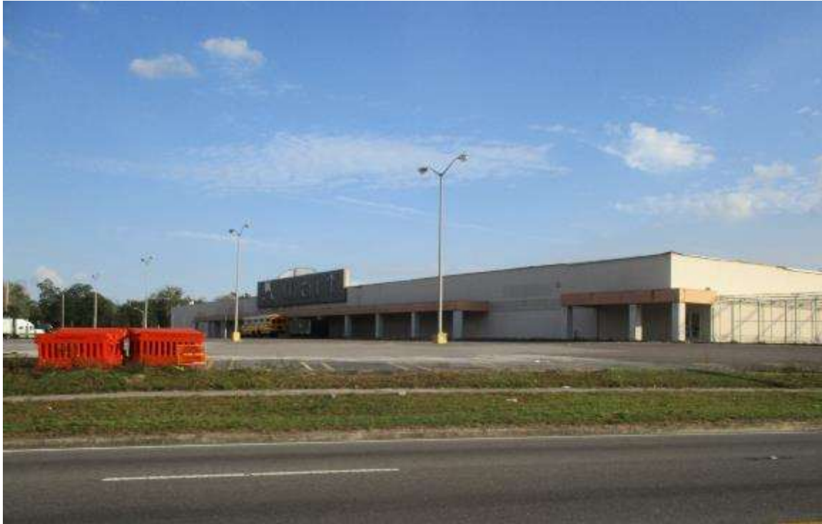
View of existing building on subject property
