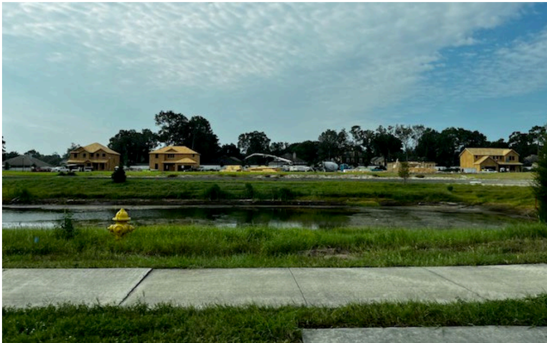
View of subject property, PUD to match adjacent single family lots
