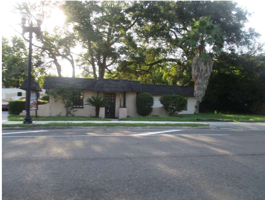
View of the Subject Site from Rogero Road
