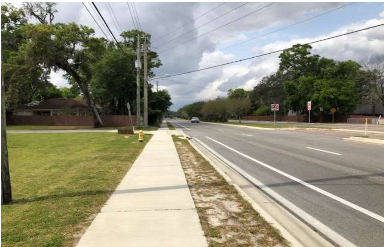
Facing west along McCormick Road from the subject site
