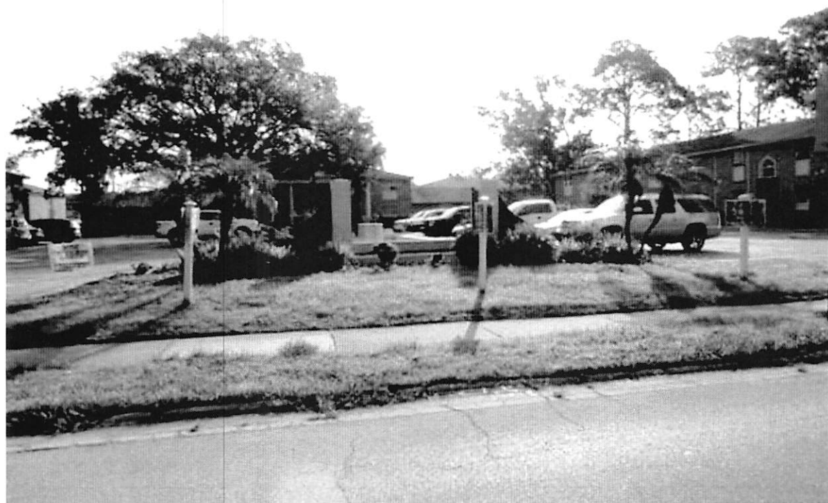
View of subject property with sign removed.
