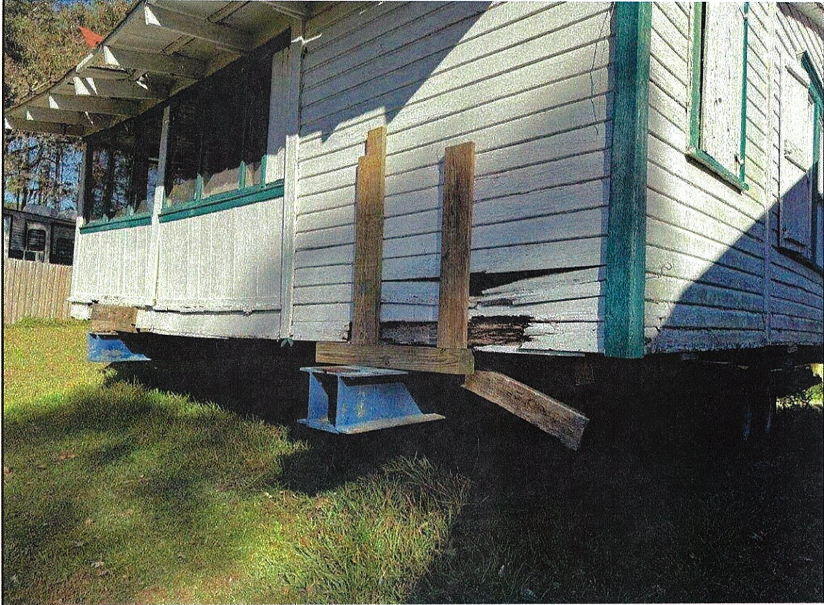
Photo 5 – House on Frame Showing Wood Frame Shoring/Repair
