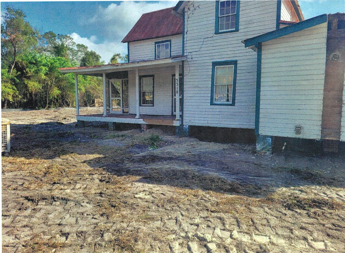
Photo 2 – Exterior of House on Brick Piers With Chimney Removed
