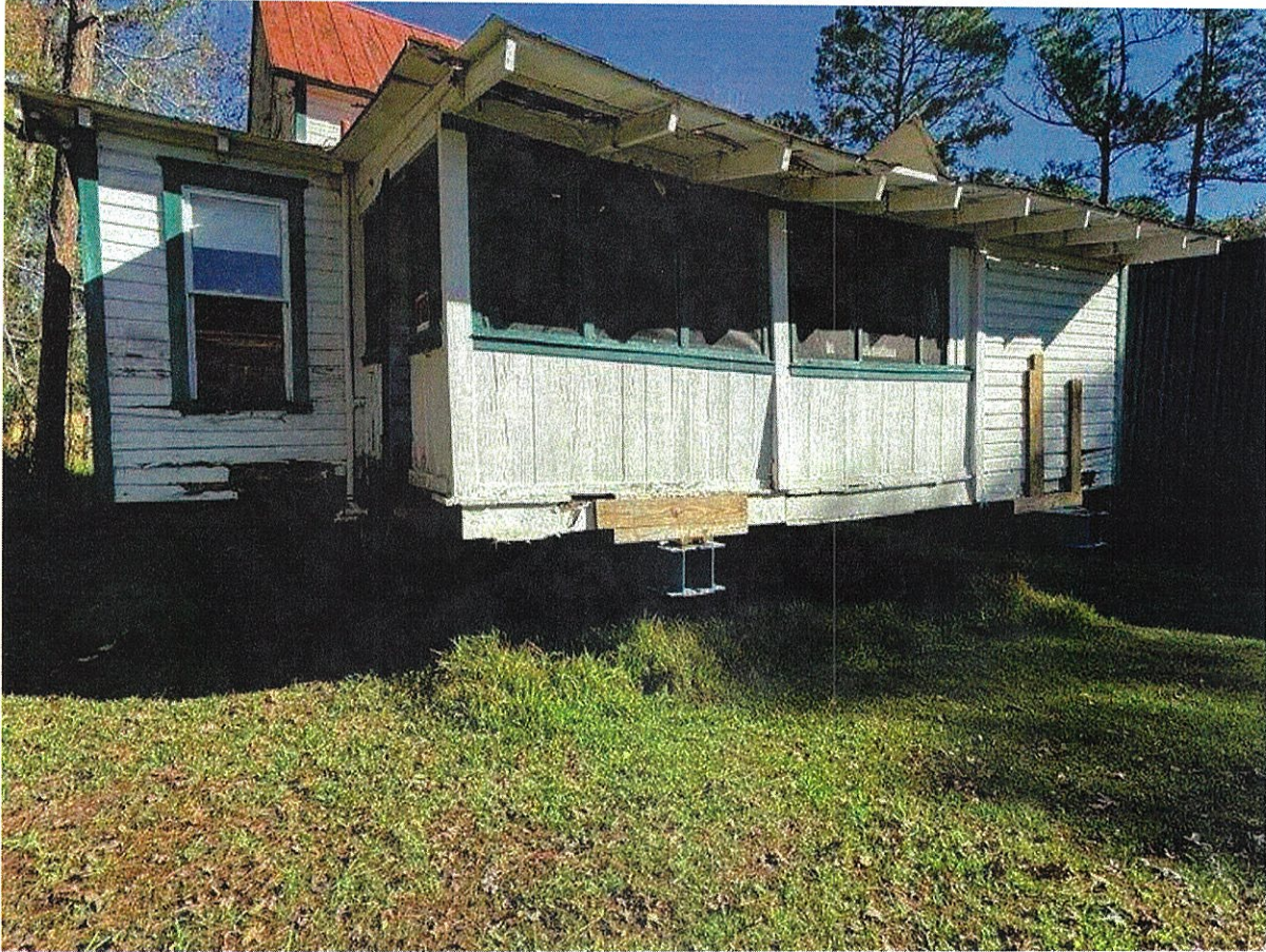
Photo 3 – Exterior of House Loaded on Steel Frame System
