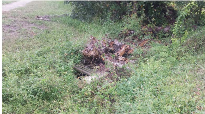
Figure 2.3 Debris Reducing Capacity of a Drainage Structure
