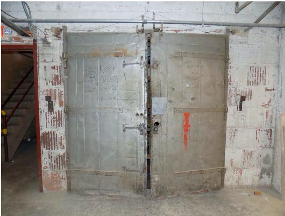
Photo 28 - Interior, basement Unit E, elevator fire shutter door, looking east.
