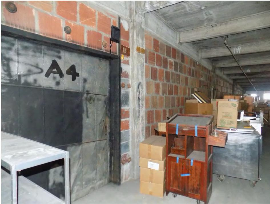
Photo 27 - Interior, fourth floor Unit A, terra cotta wall and automatic fire door, looking west.
