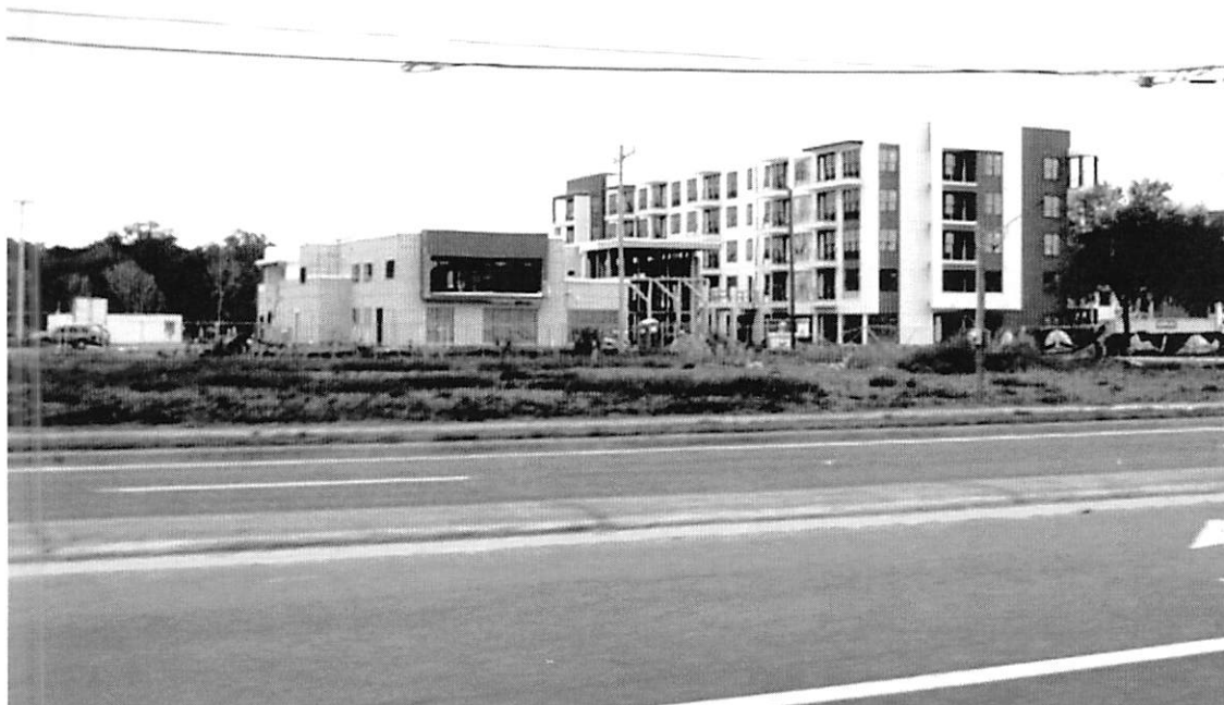
New multi-family dwellings under construction
