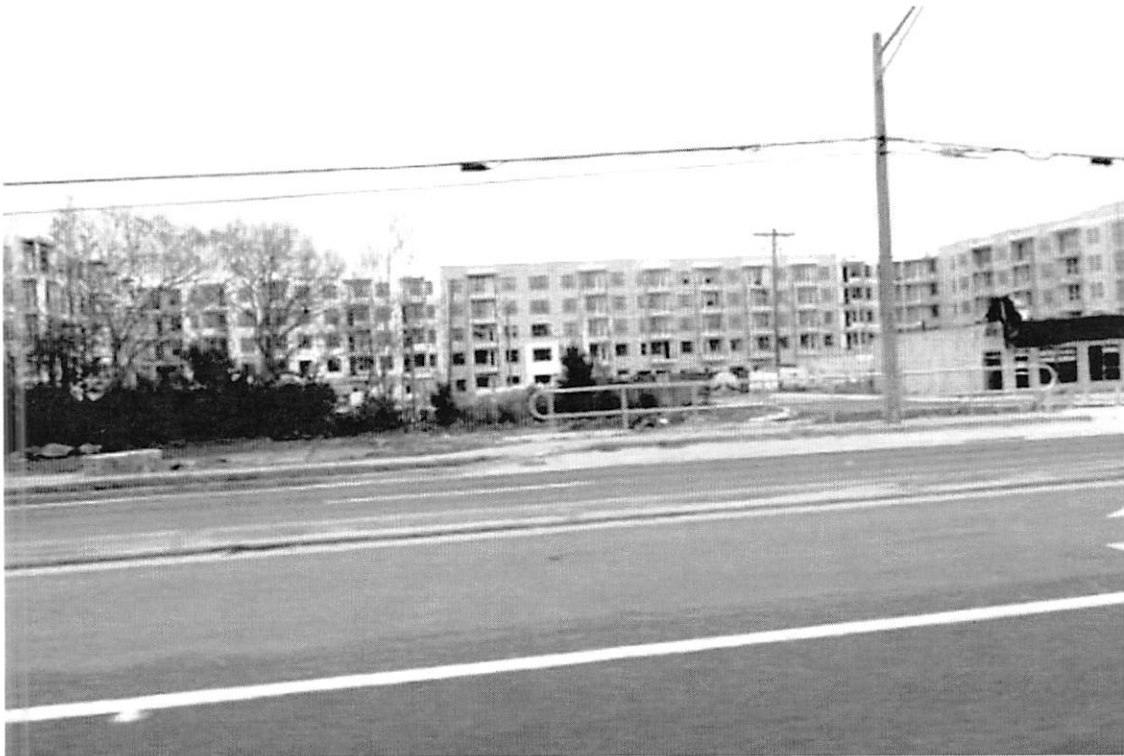
New multi-family dwellings under construction
