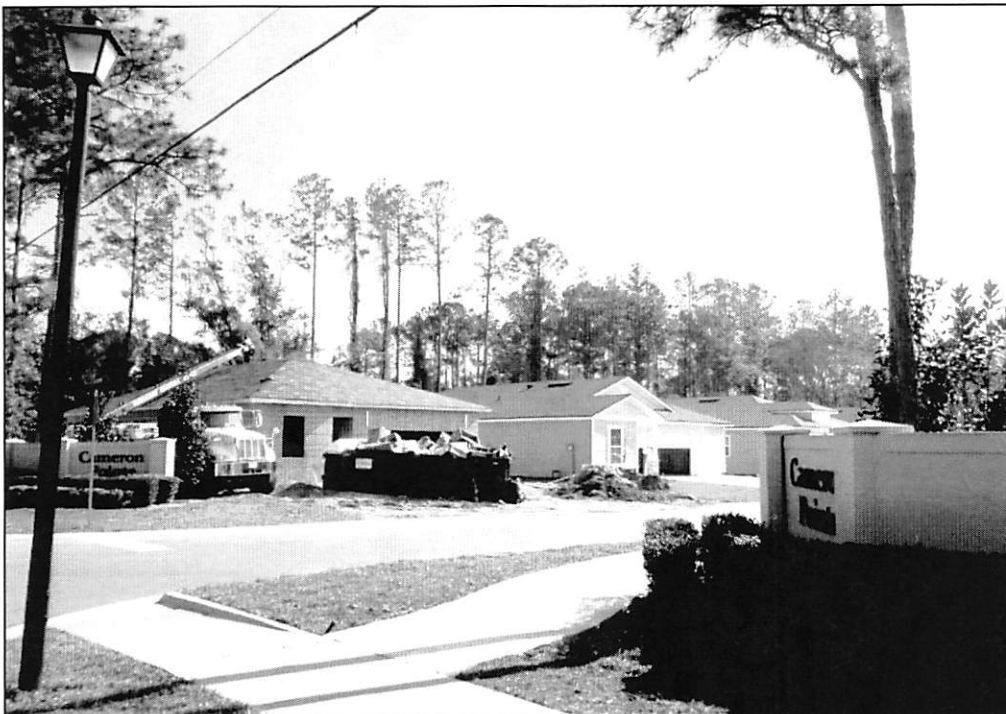
View of Subdivision to the South Cameron Pointe
