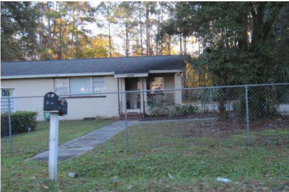
Adjacent single family dwelling dwelling
