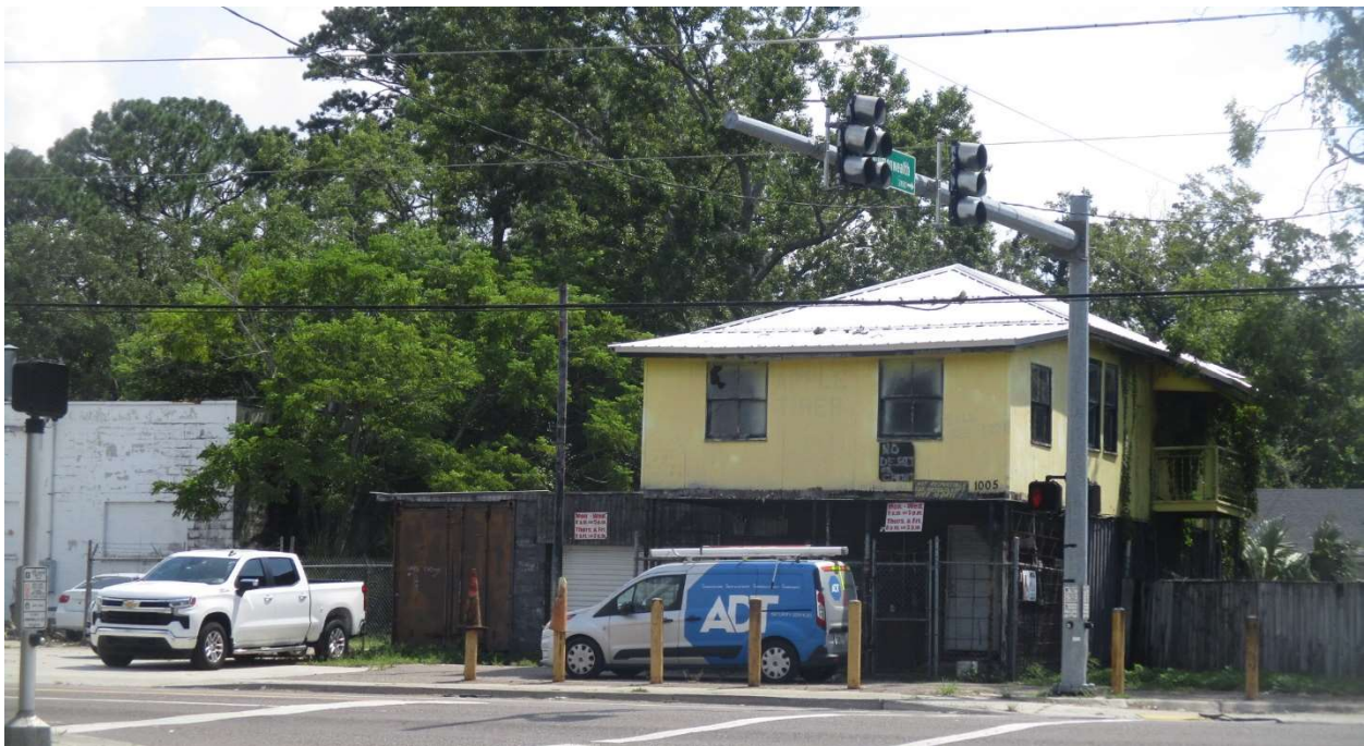
Source: Planning & Development Department, 8/14/24
