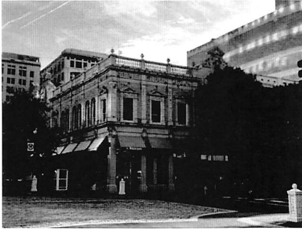
Figure 4-Current View of the Old Bisbee Building
