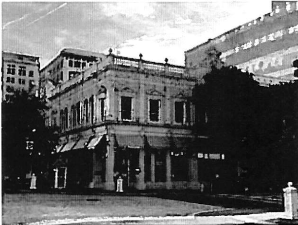
Figure 6-Current View of the Old Bisbee Building
