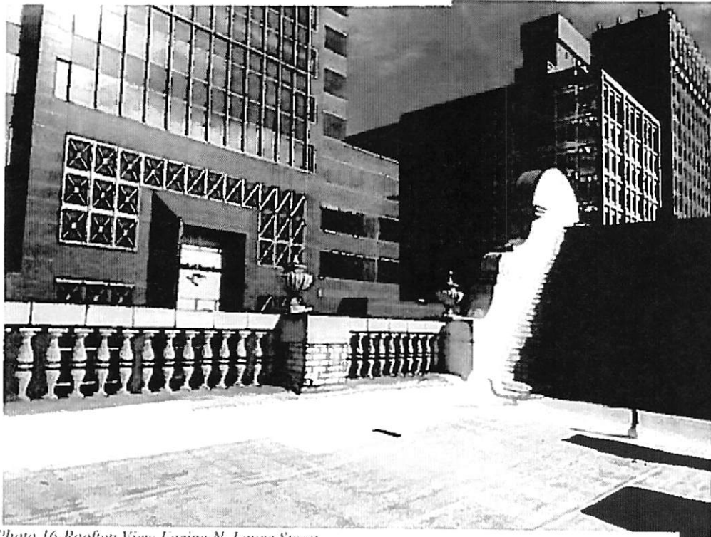
Photo 16-Rooftop View Facing N. Laura Street
