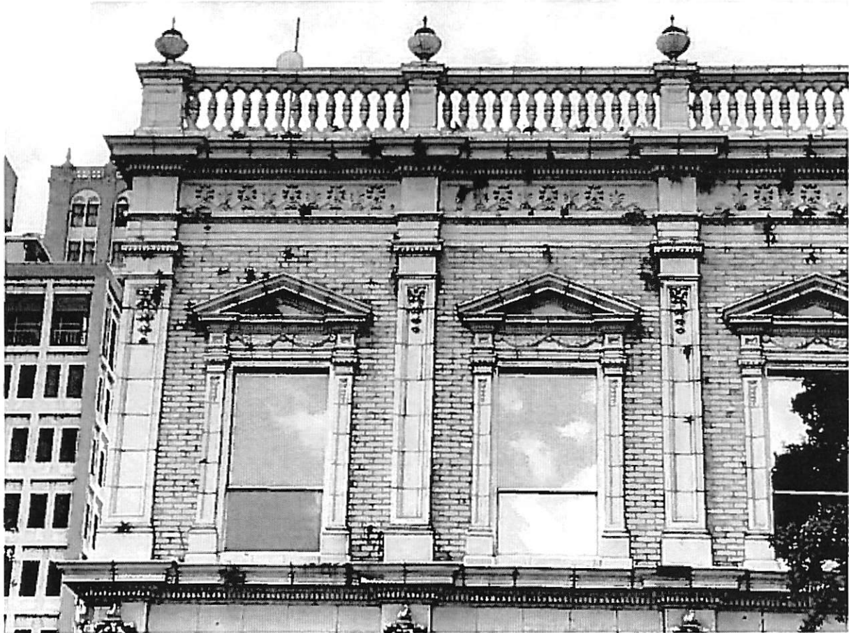
Photo 12-Close-up of the Second Floor Along W. Bay Street
