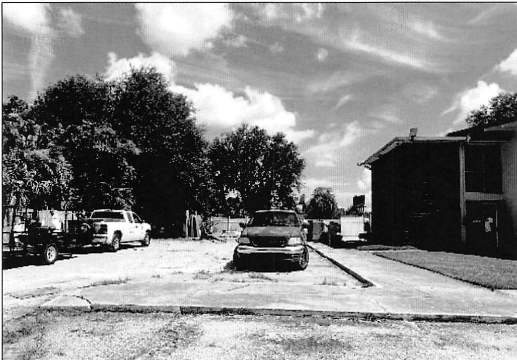
View of Existing Parking 6545 Ramona Blvd.
