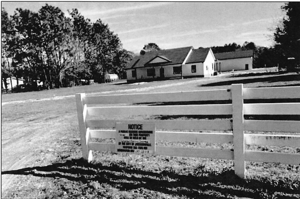
Subject Property: 1221 Cathy Tripp Lane North
