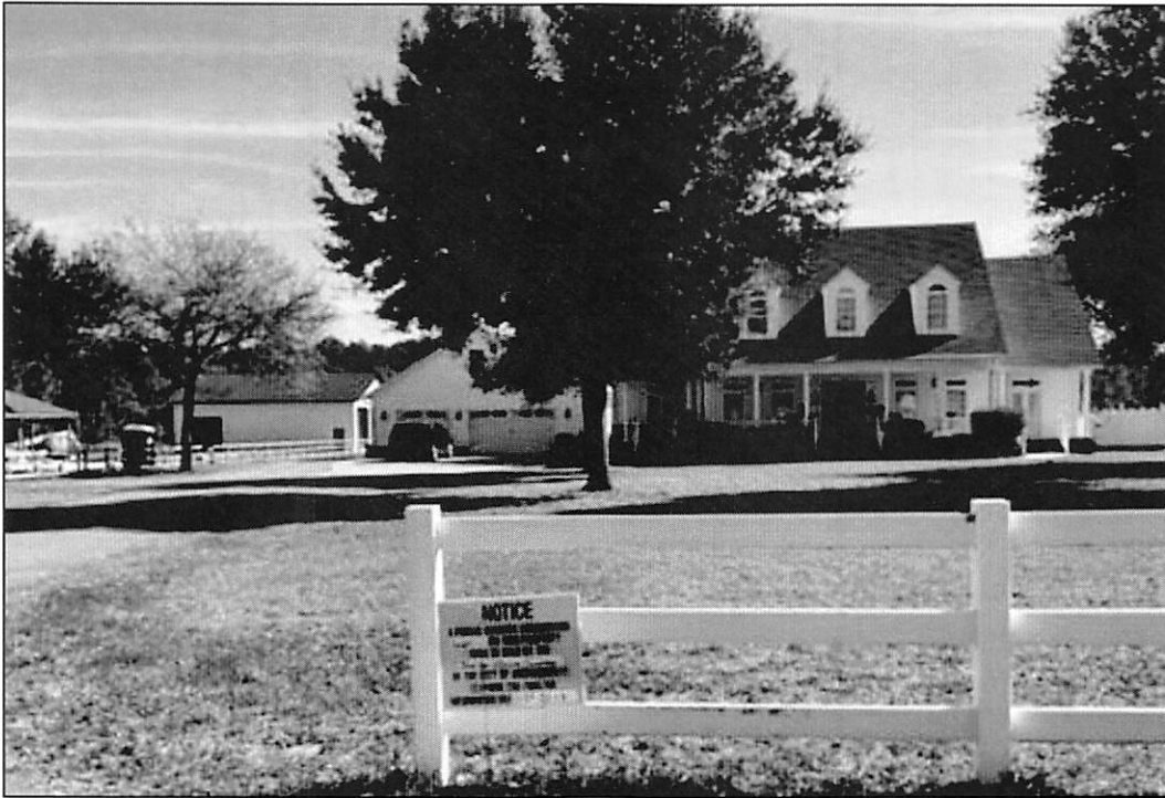
Subject Property: 1229 Cathy Tripp Lane North
