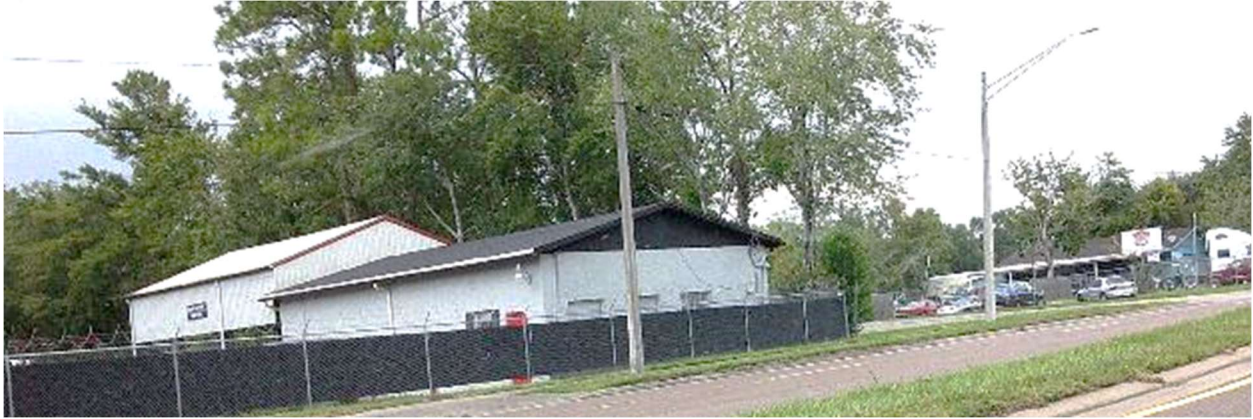
View of properties opposite of subject property
