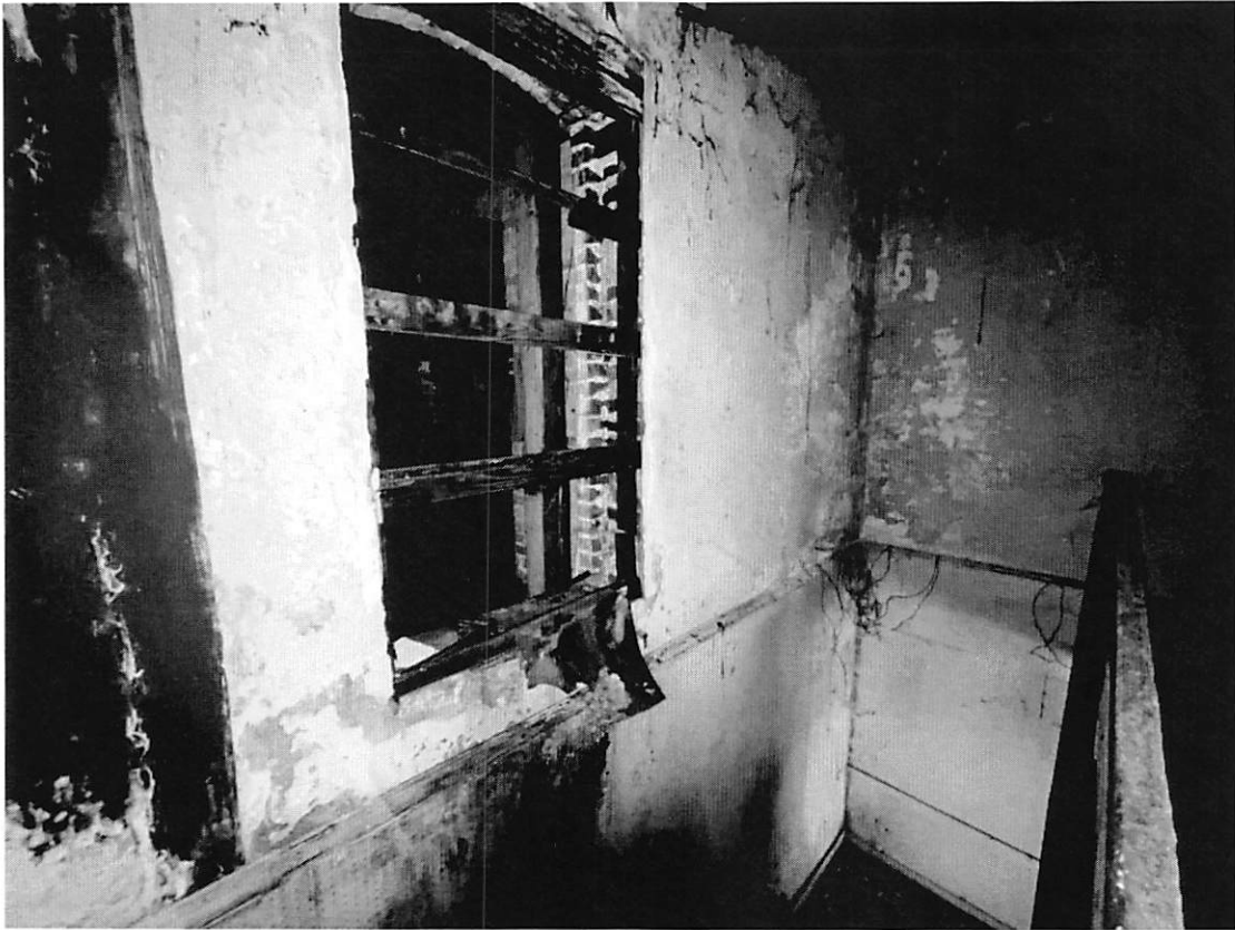
Top of stairs, rear northwest corner
