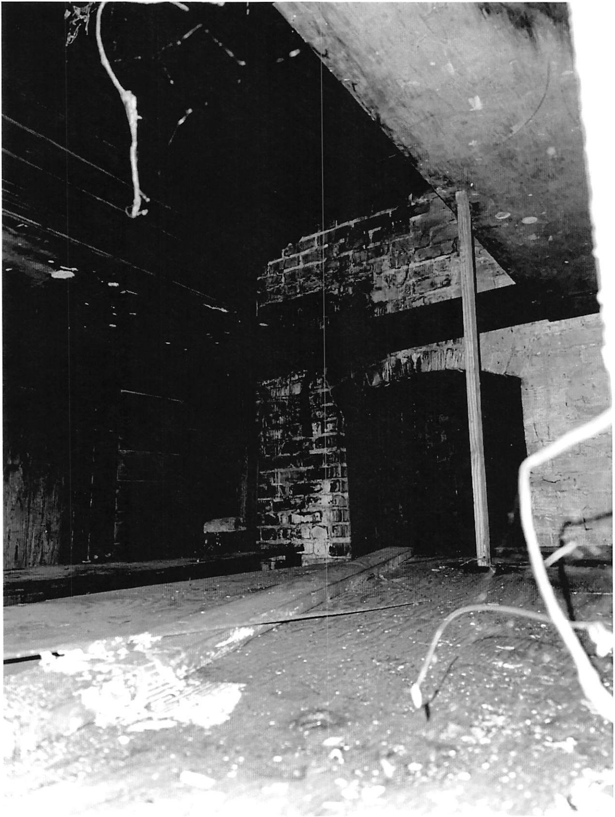
Upstairs, porch detail
