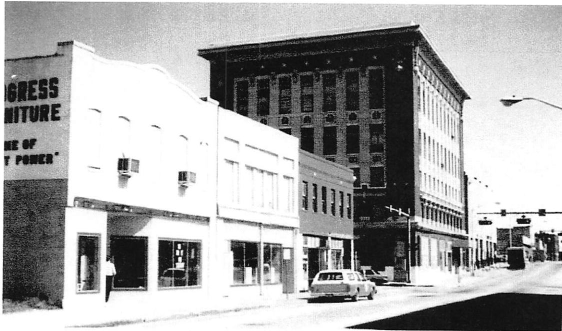
318 North Broad Street during the early 1990s. Photograph courtesy of the City of Jacksonville.
