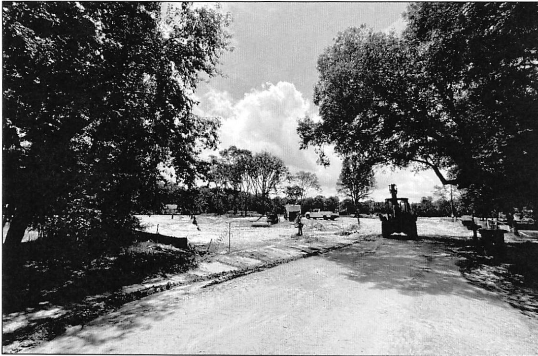
View of Property to the South (Jacks Road PUD)
