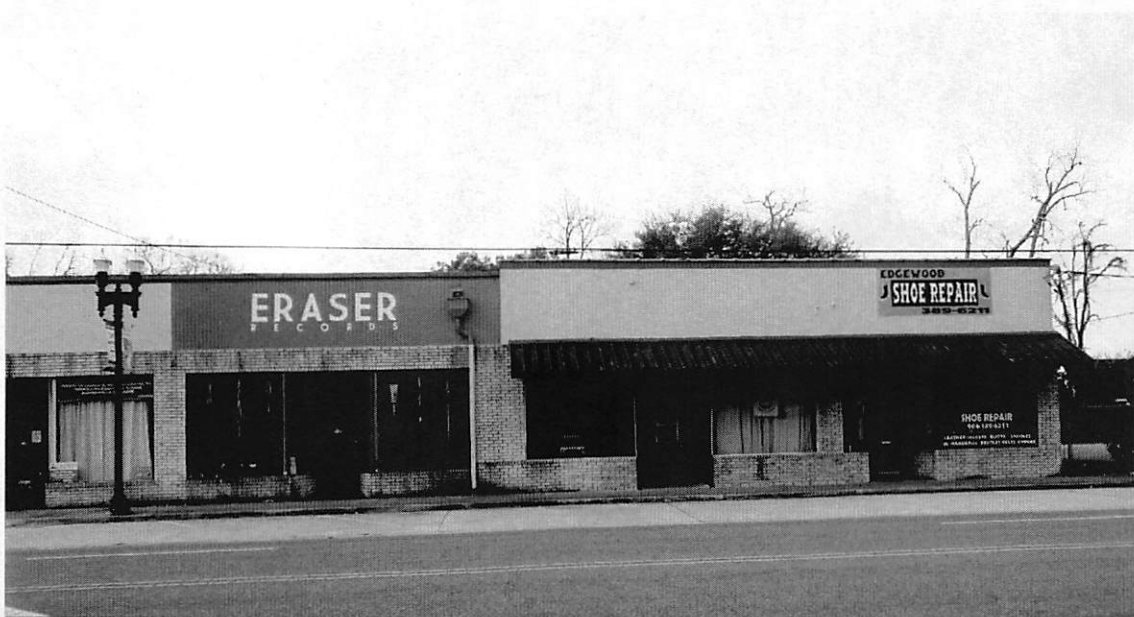
Property across Edgewood Avenue: Commercial Shopping Center
