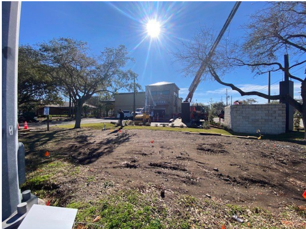
View of the Subject Site from Beach Boulevard
