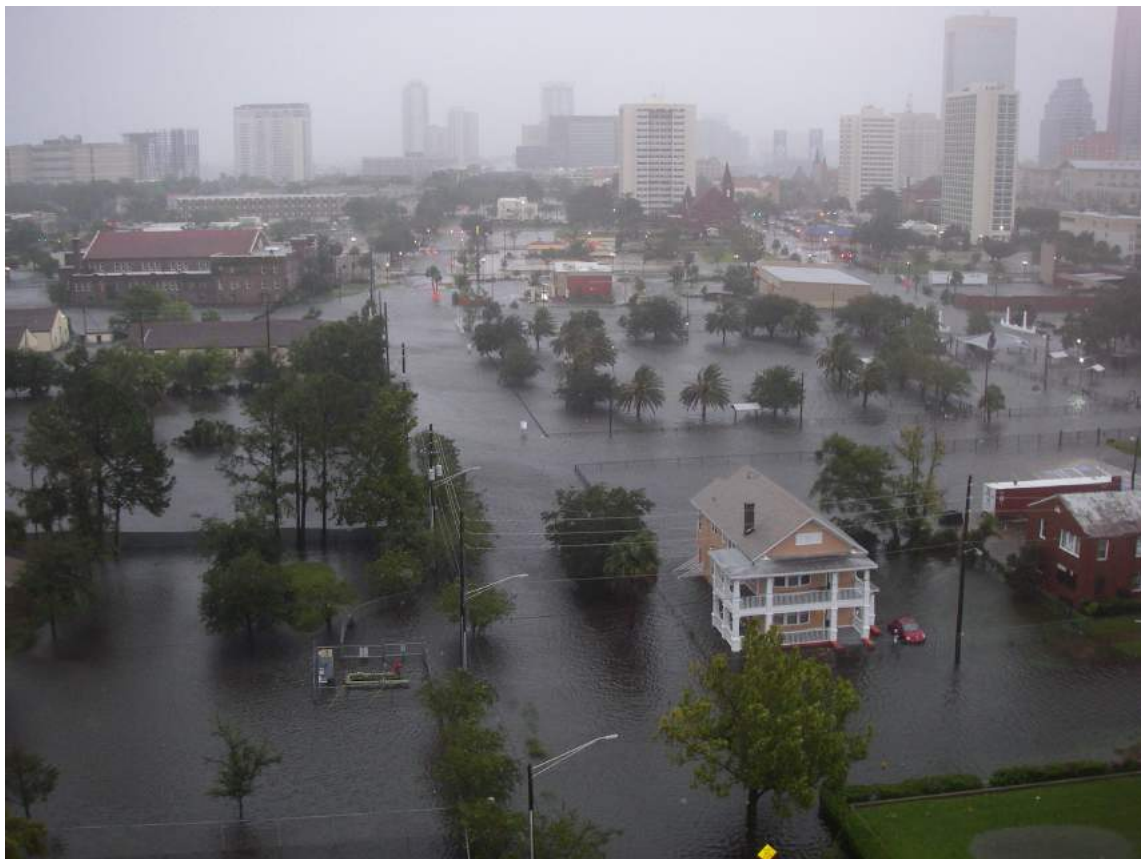
Springfield Flooding from Hurricane Irma in 2017
