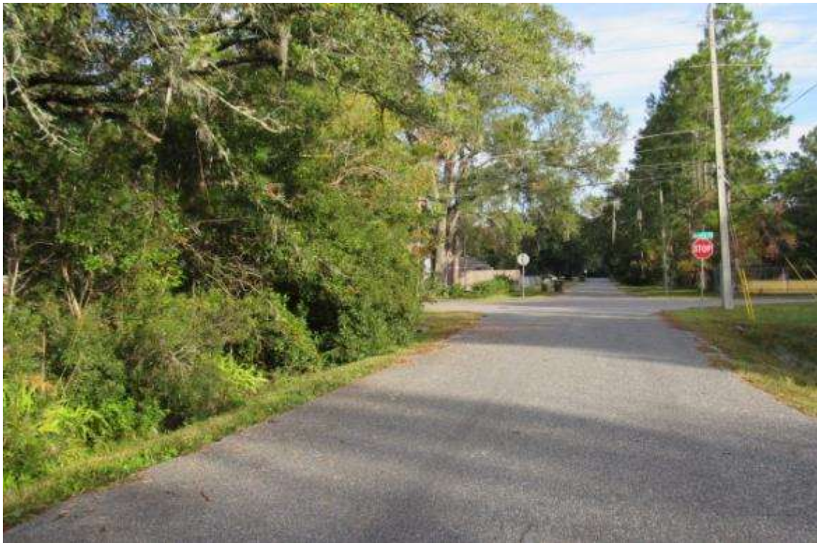
Navaho Road with drainage swales on each side.
