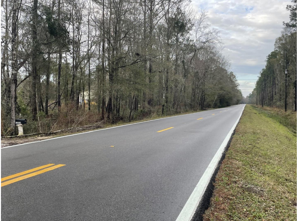
Source: Planning & Development Department, 1/24/2024
