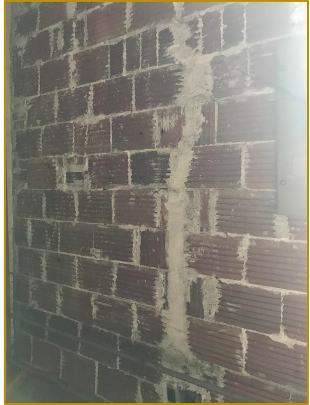
Figure 8-Original red terracotta brick exposed in the building's current condition
