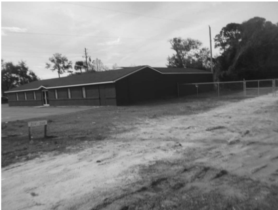
View of the neighboring office building to the south.
