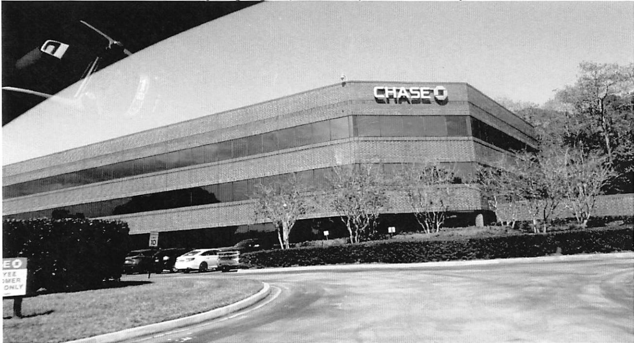
View of subject property from Baymeadows Way West.
