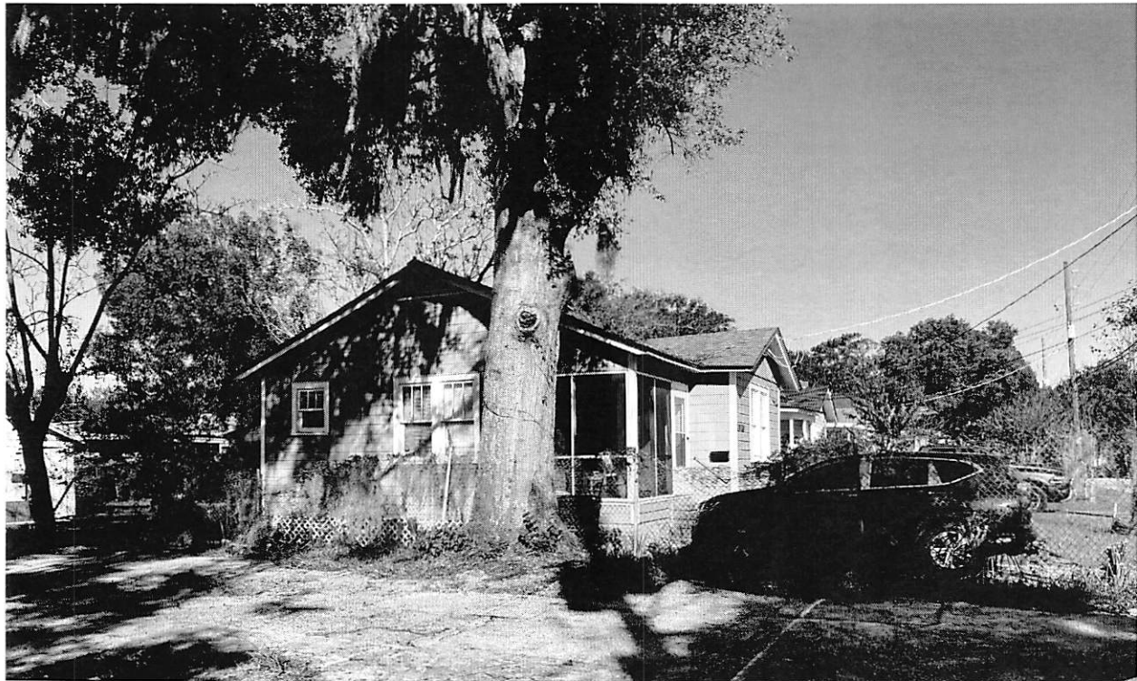
Property to the North: Single Family Dwelling
