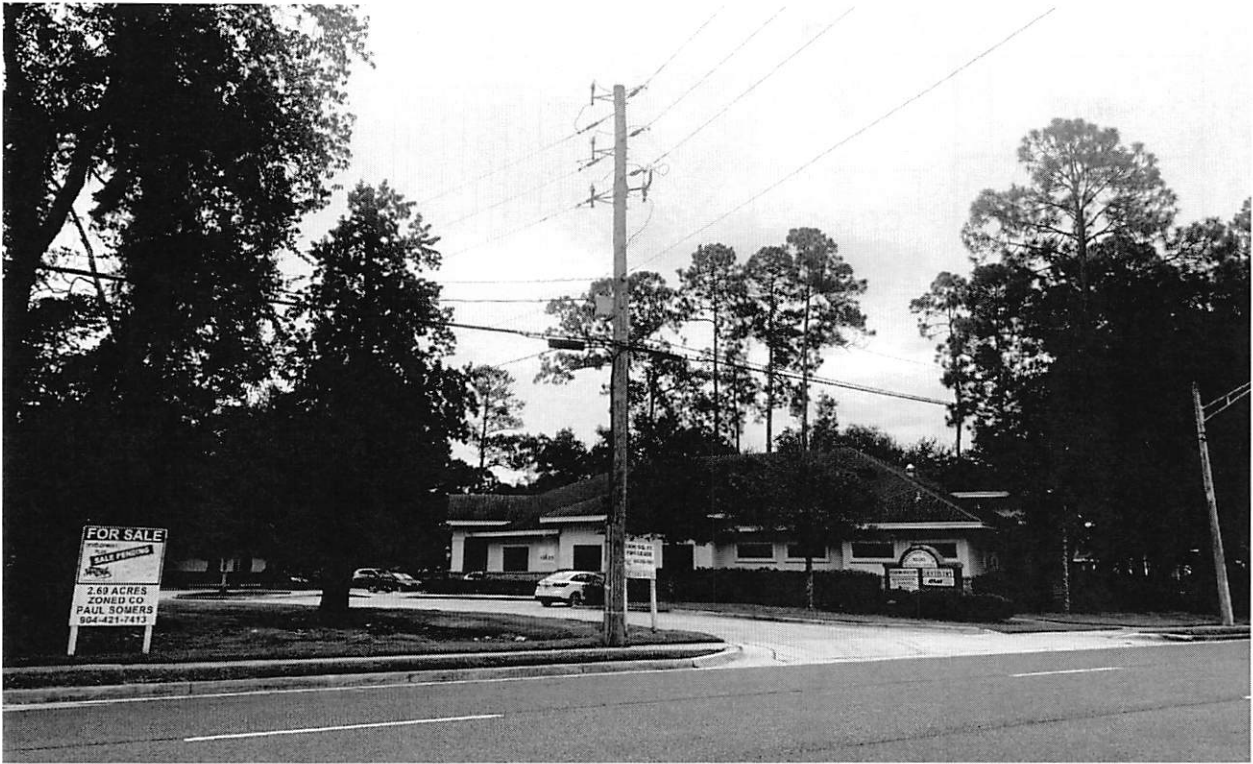
Source: Planning and Development Department, 8/20/20 View of commercial offices, south of subject property.
