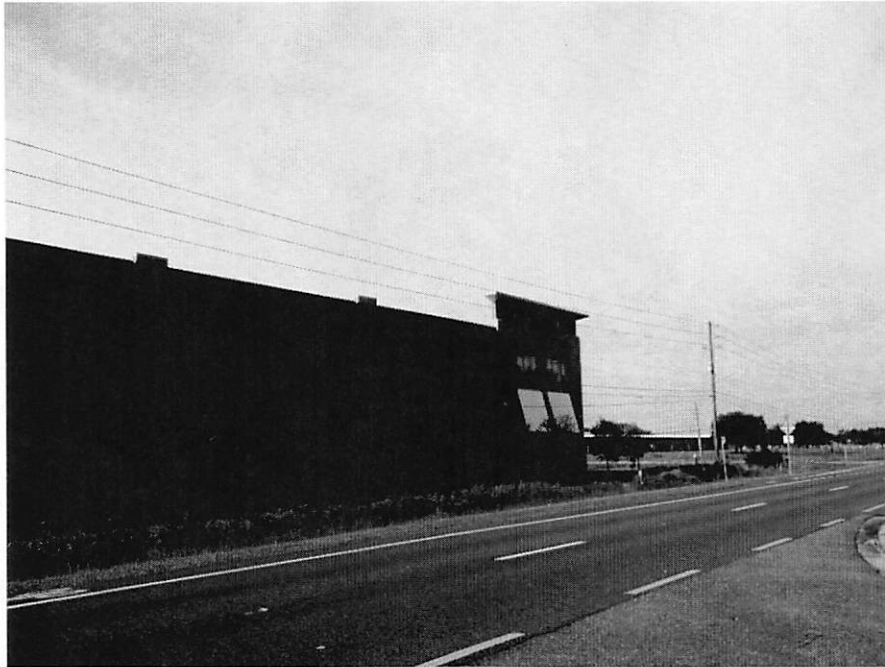
View of the Storage Facility across Normandy Boulevard from the Subject Site.
