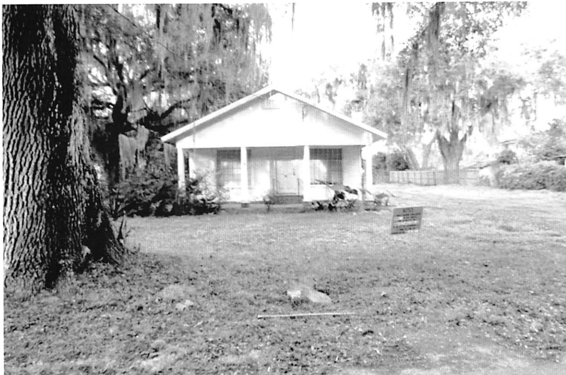
Existing dwelling to be removed.
