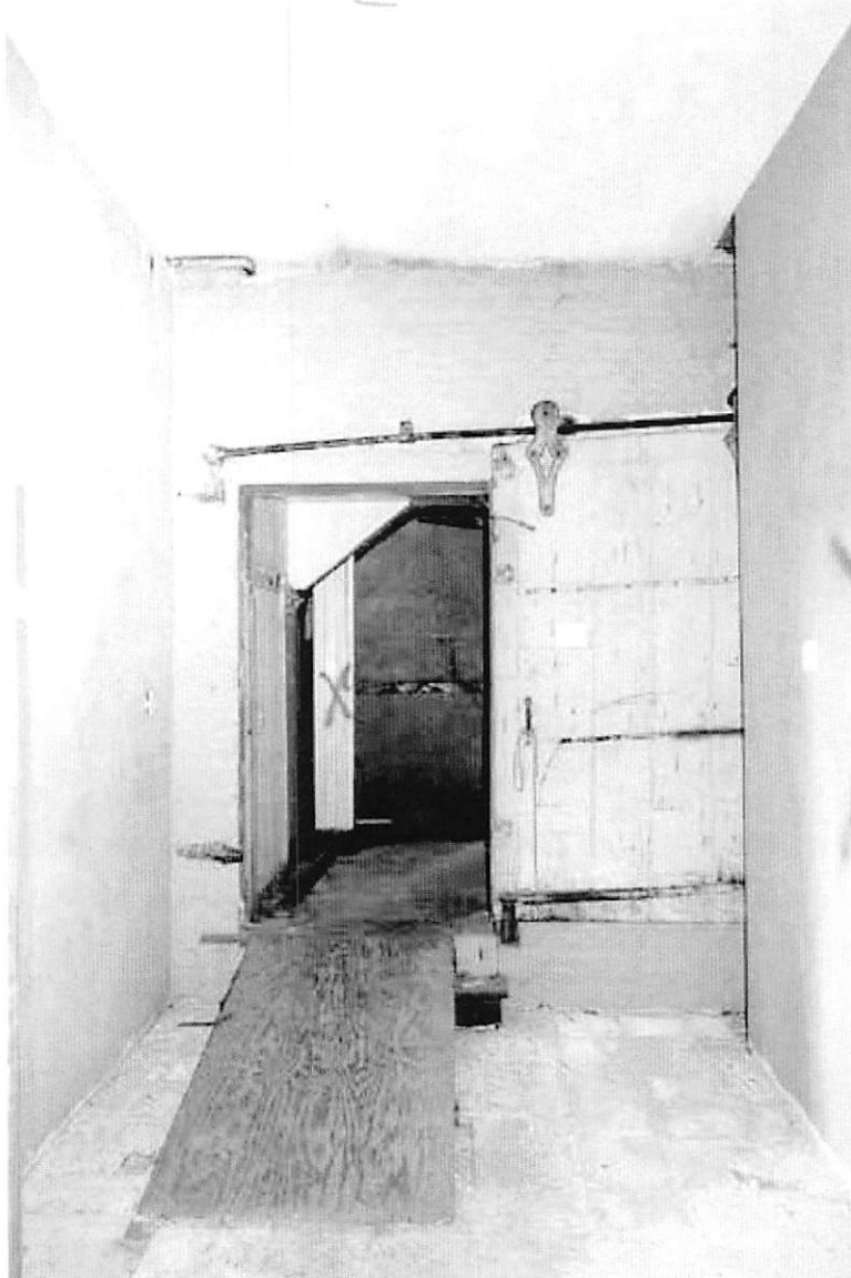
12 of 28: Detail of typical fire door; photographer facing southwest.
