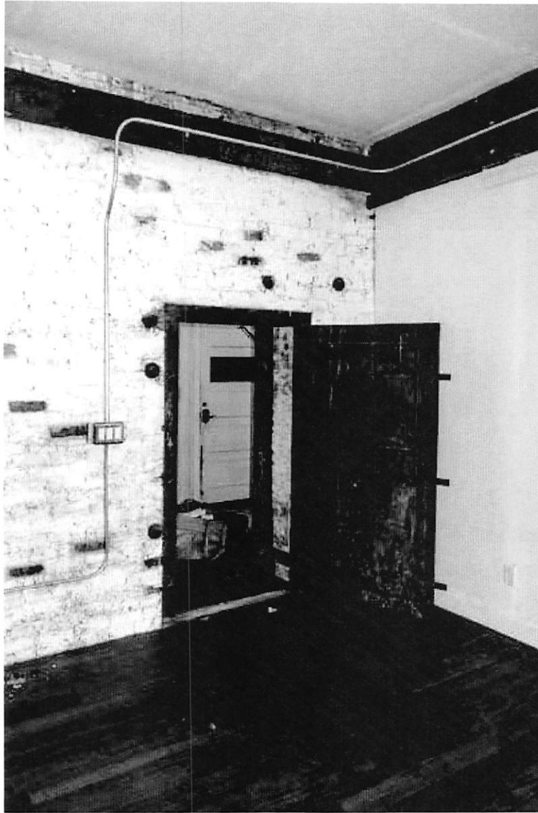
27 of 28: Detail of another historic fire door found on second floor; photographer facing east.
