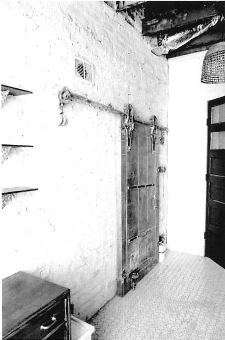
24 of 28: Detail of typical historic fire door of second floor; photographer facing east.
