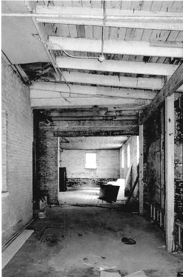
8 of 28: Interior view along covered drive to garage; photographer facing northeast.
