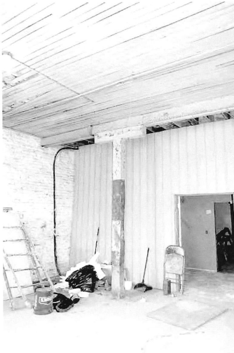
11 of 28:Detail of typical support post of garage; photographer facing southwest.
