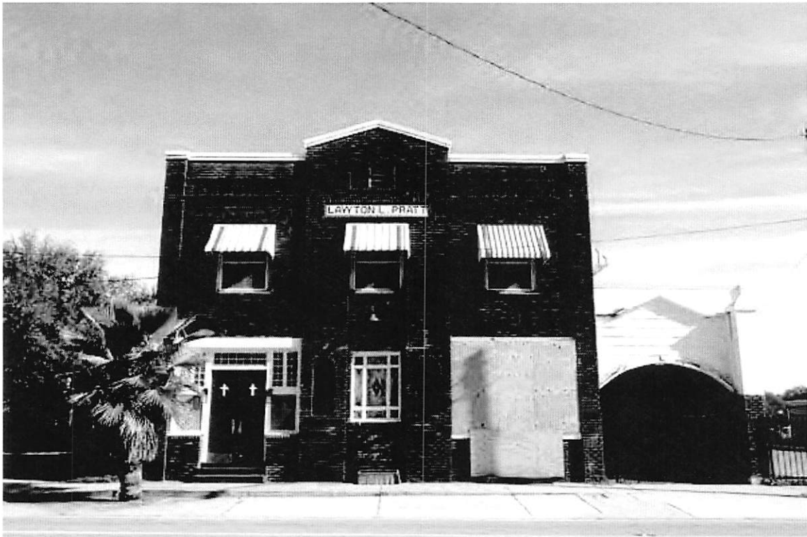
2 of 28: South front elevation; photographer facing northeast.
