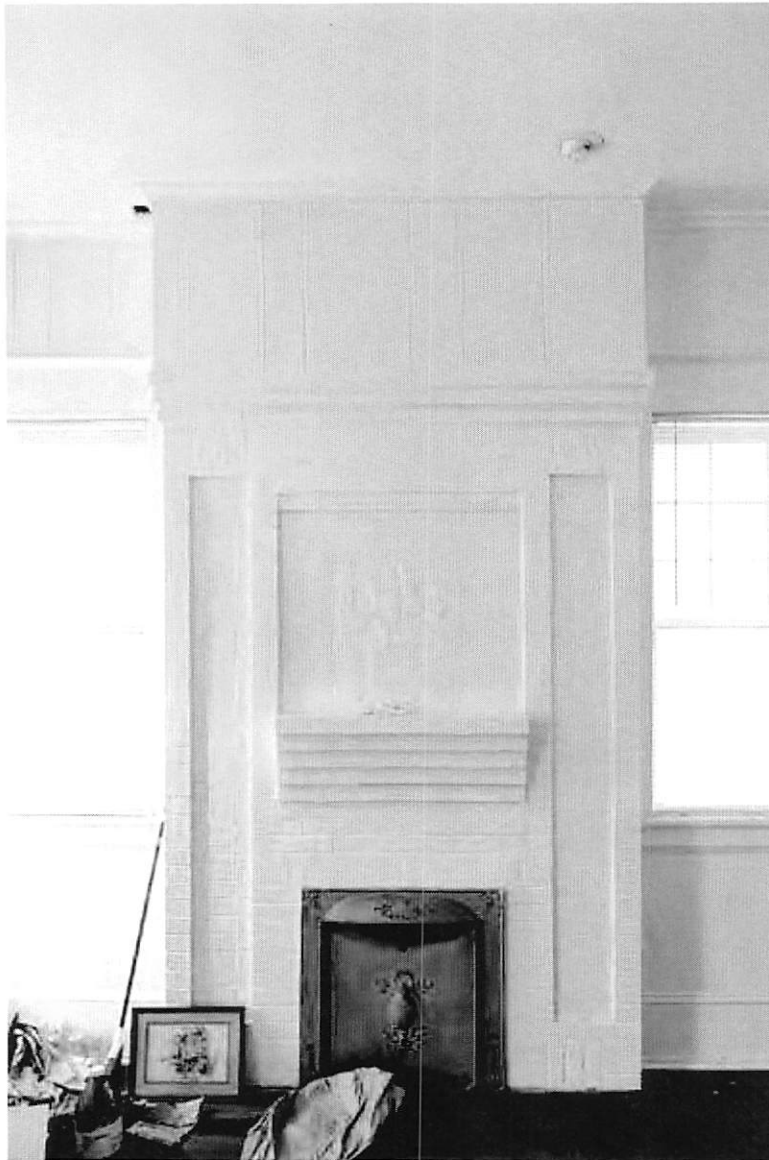
16 of 28: Detail of fireplace in foyer before chapel; photographer facing northwest.
