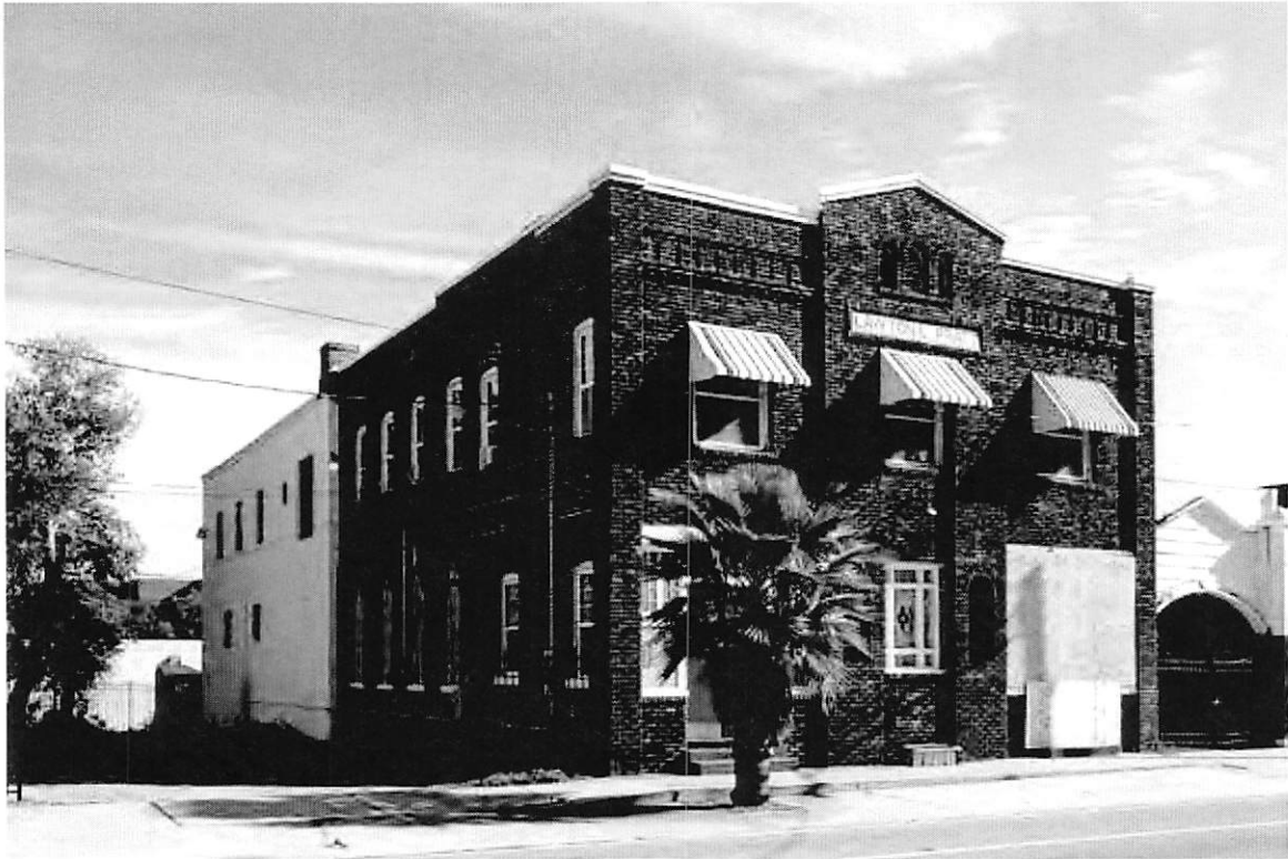
1 of 28: Oblique view of the west side and south front elevations; photographer facing northeast.
