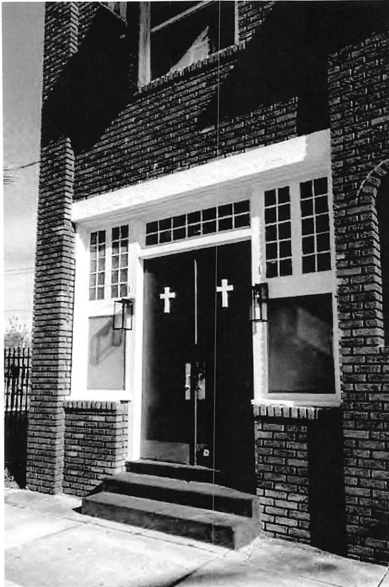
4 of 28: Detail of front entrance, photographer facing northwest.
