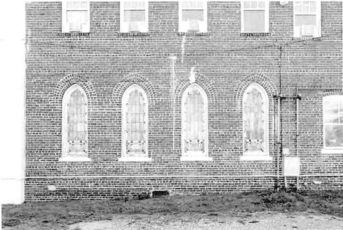
7 of 28: Detail of stained glass windows of chapel; photographer facing southeast.
