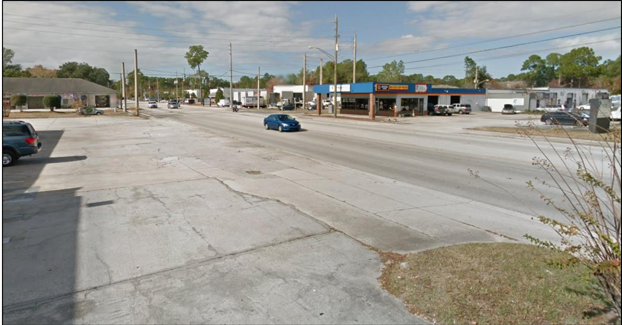
Existing Driveway access along Sunbeam Road
