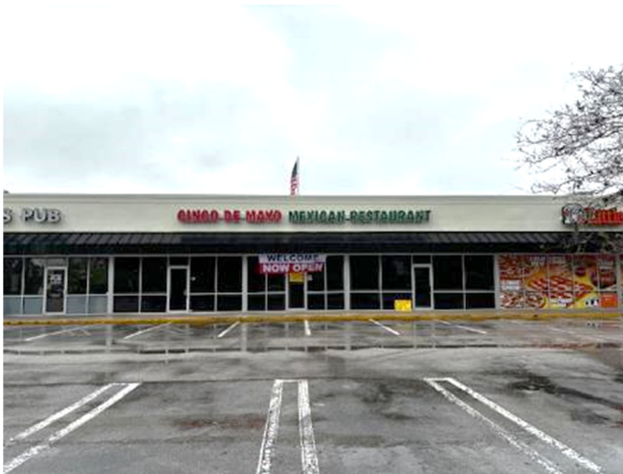
View of Subject Restaurant Seeking Exception Source: Planning and Development Department November 17, 2023
