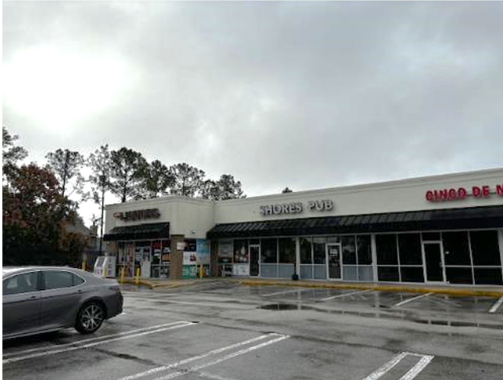
View of Adjacent Pub Serving all Alcohol Source: Planning and Development Department November 17, 2023
