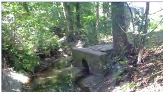
Major Outfall, City of Jacksonville Public Works
