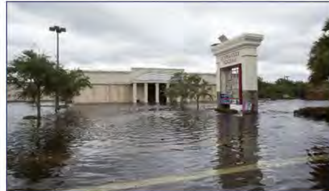
Hurricane Irma – Roosevelt Square Shopping Center, September 11, 2017
