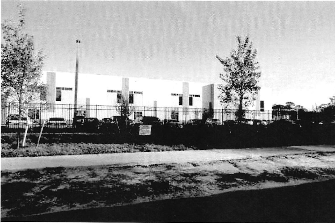
School under construction
