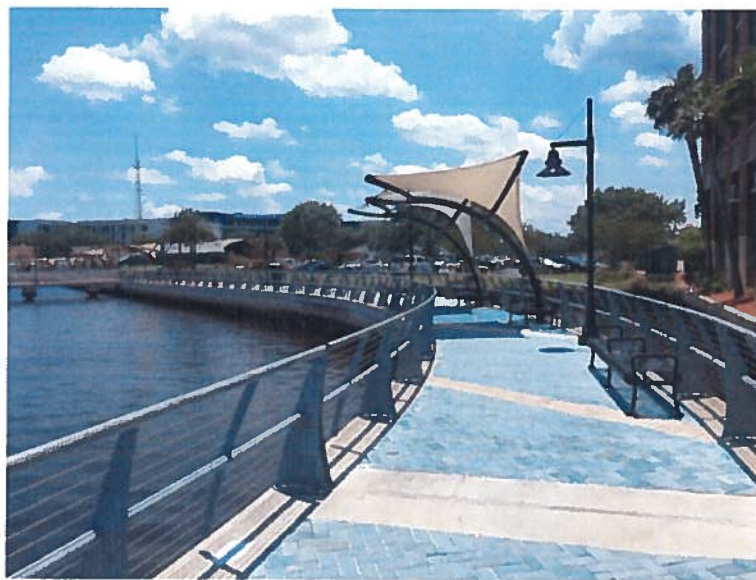
Existing Southbank Riverwalk railing and materials.
